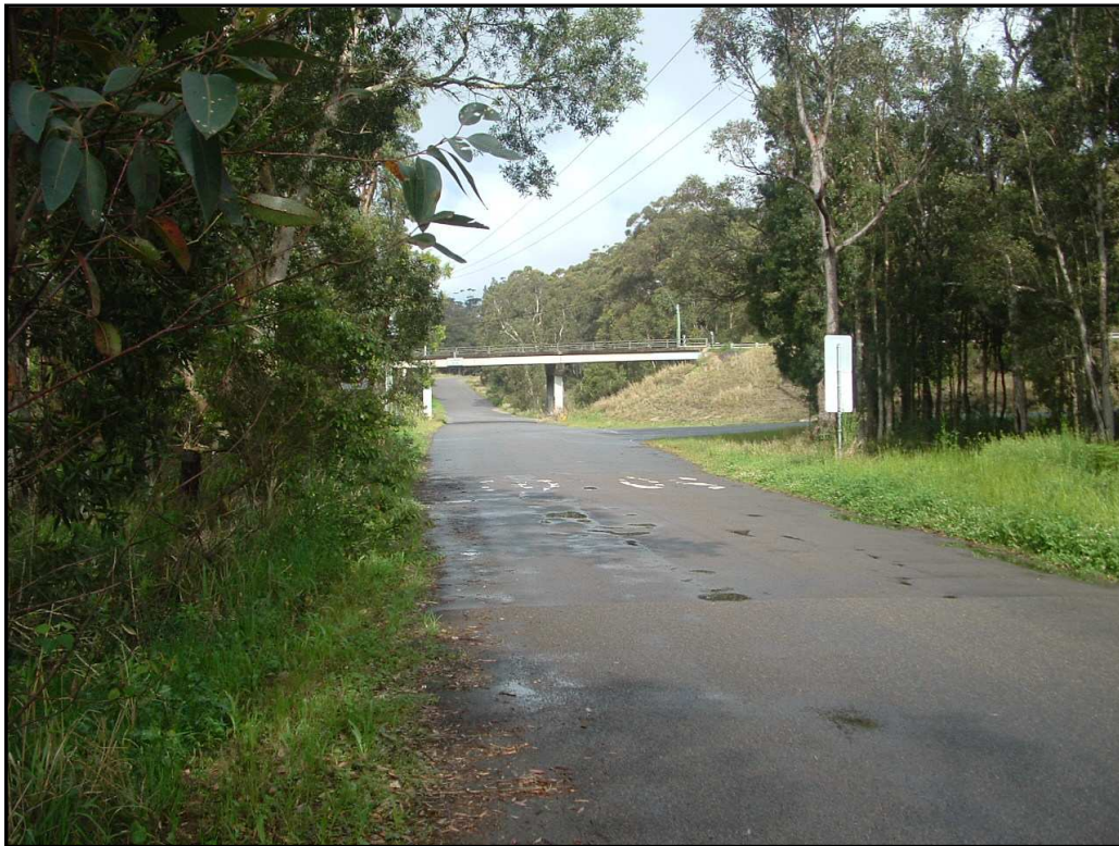
Photo 5 – View east (left) for vehicles exiting site access
