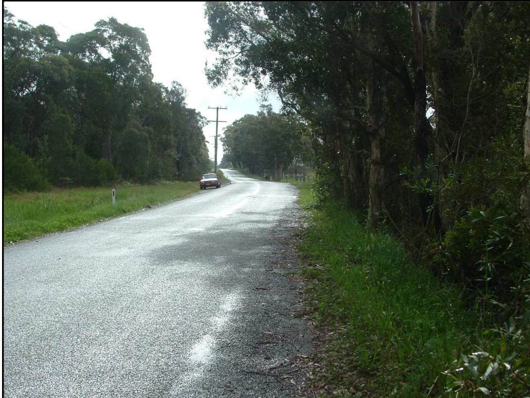
Photo 4 – View west (right) for vehicles exiting site access
