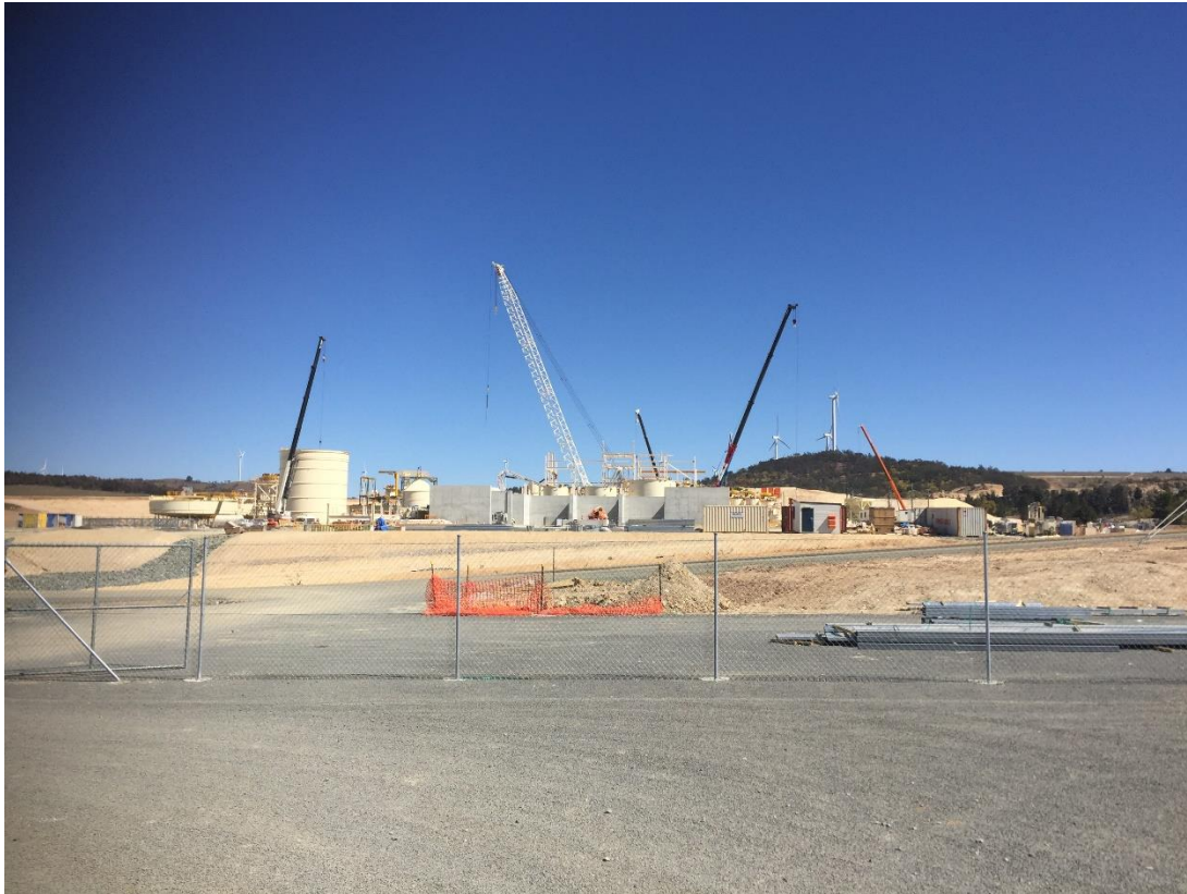
9. Construction of TSF4 – facing north west.
