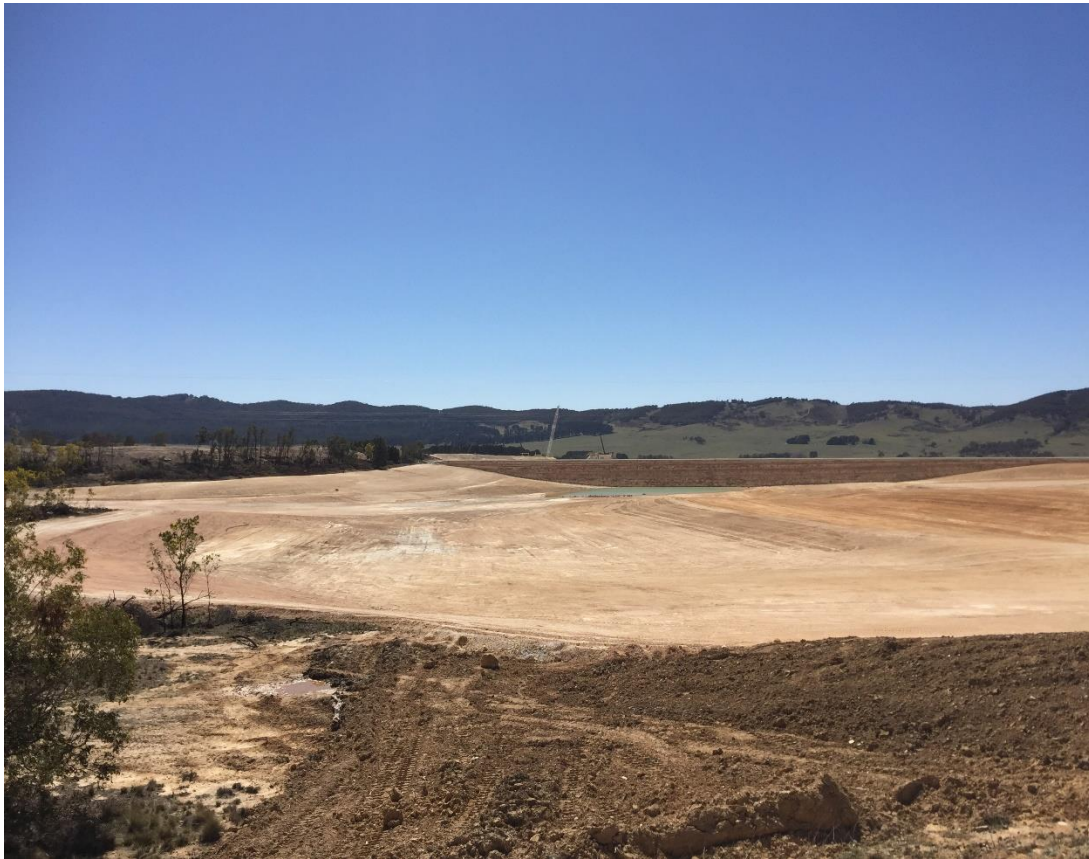
1. View of proposed Tailings Storage Facility (TSF4) facing north.
