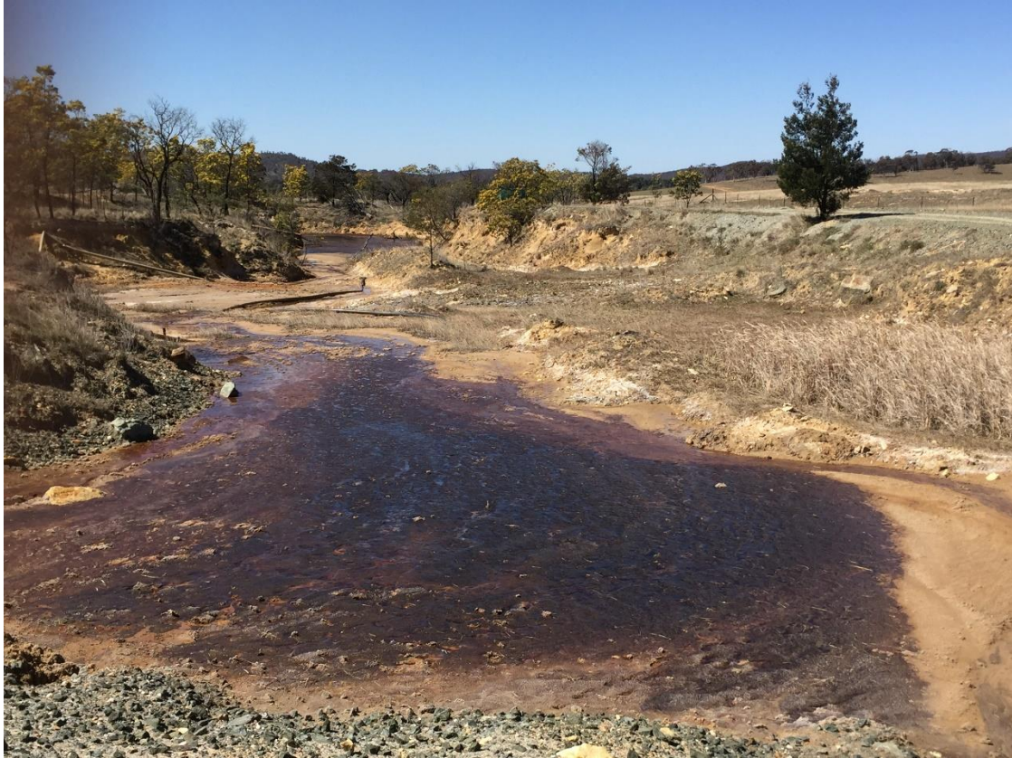
3. Seepage evident south of Tailings Dam South (TDS).
