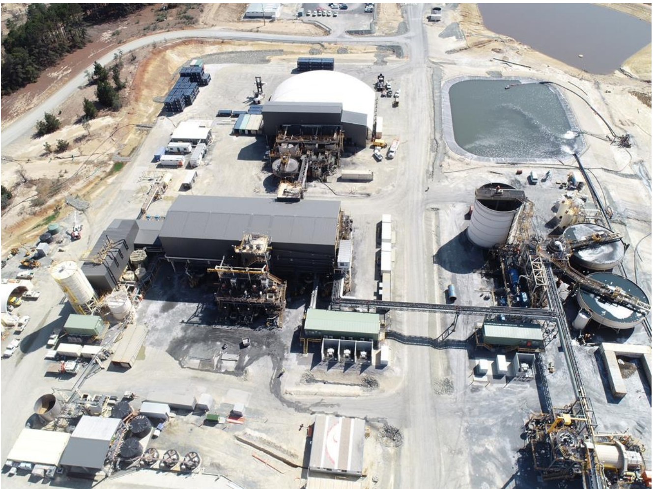
Figure 1. Overview of the completed processing plant - January 2020
