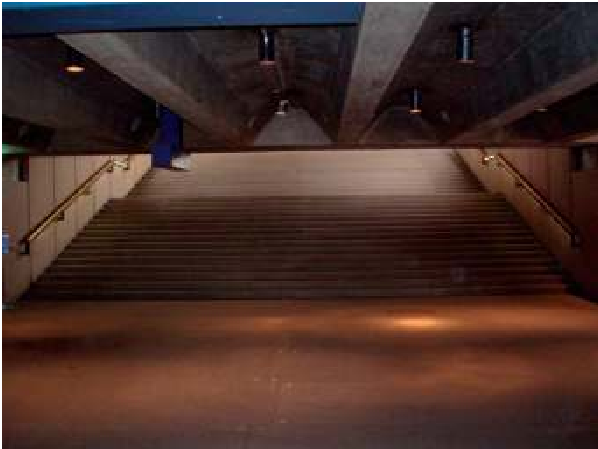
Figure 5: Existing Concert Hall stairs viewed from Box Office Foyer Level
