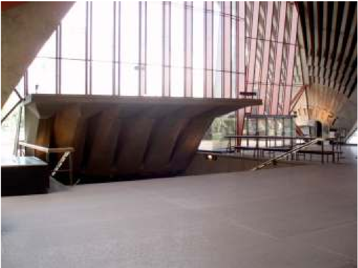
Figure 7: Existing Concert Hall stairs viewed from Southern Foyer Level
