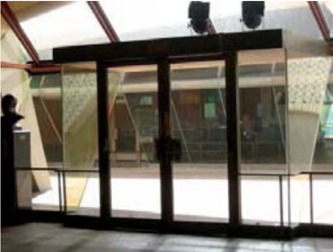
Typical existing Level 42 Southern Foyer egress door
