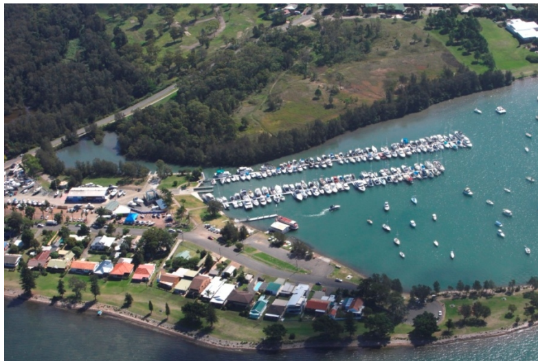
Illustration 10 – The existing Marmong Point Marina from East
