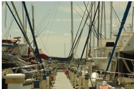
Illustration 9 – Existing Marmong Point Marina Pontoons
