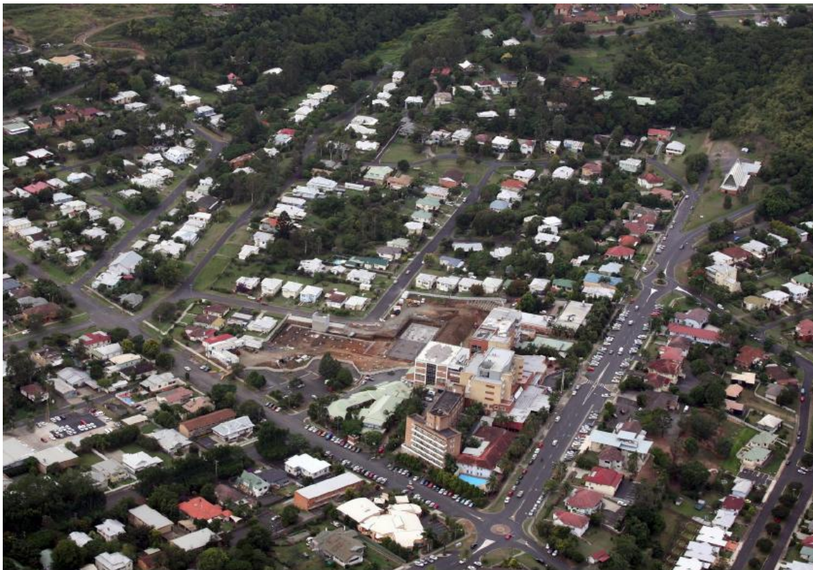
Figure 06 Lismore Base Hospital aerial photo
