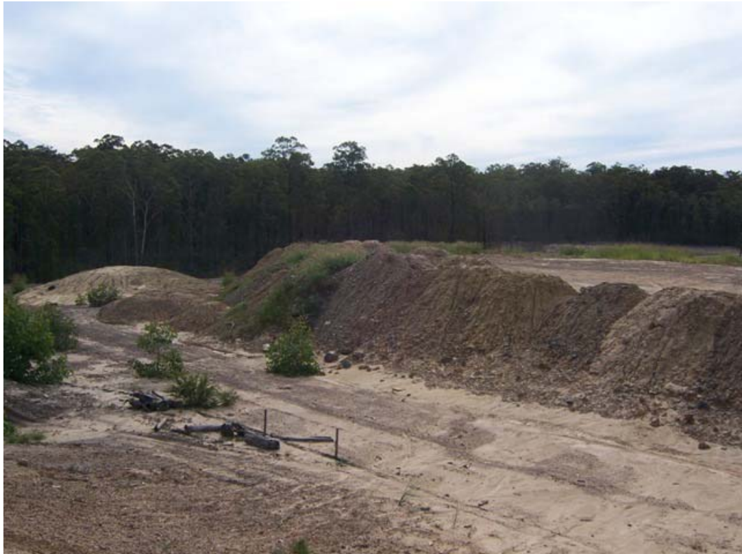
Photographs 7: Facing the North West along the northern site boundary shows fill materials assumed from the main road construction, currently stored on the north western portion of the site.
