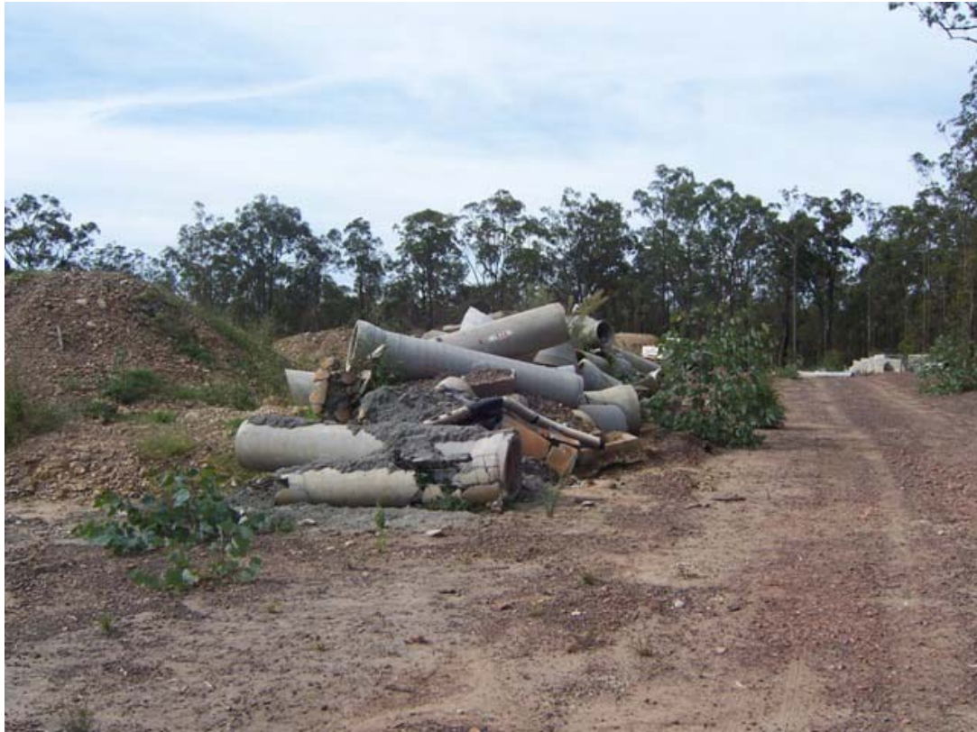
Photograph 10: Road Construction materials placed on the north western portion of the site.
