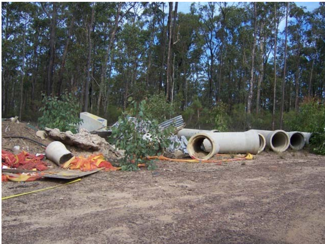
Photograph 10: construction materials and associated wastes present in the north western portion of the site.
