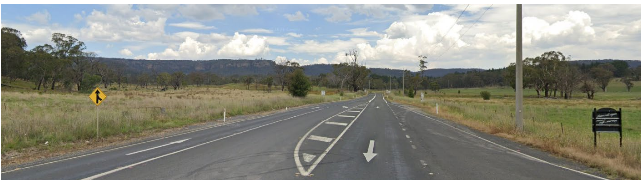
Plate 5.2 Existing advance intersection warning signage north of Castlereagh Highway/Cullen Valley Mine Access Road intersection
