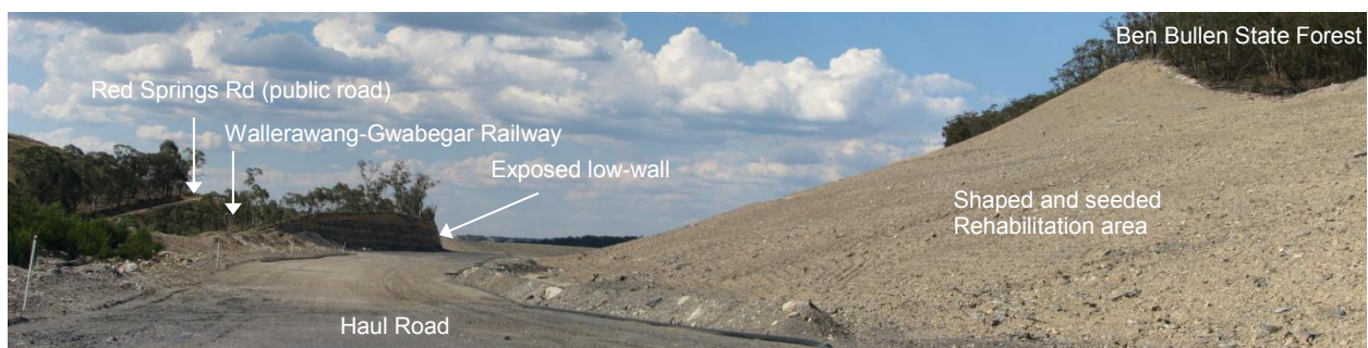
Plate 2 Void 105 - Cullen Valley Mine, looking north
