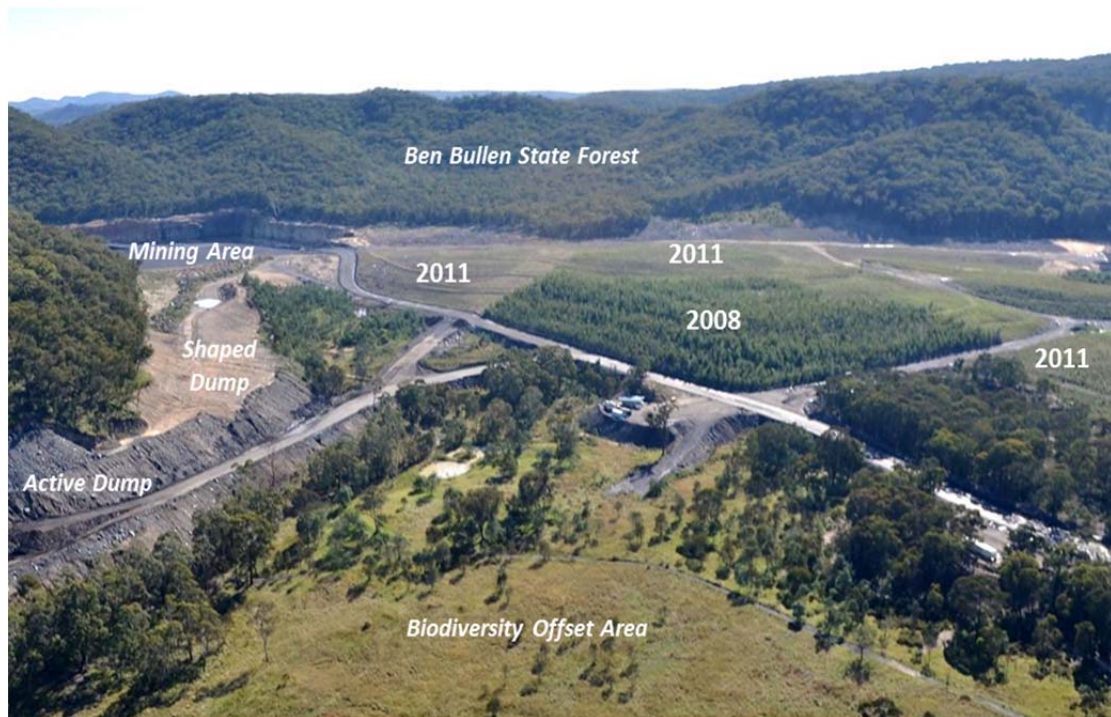
Plate 2 Progressive Rehabilitation at Invincible Colliery
