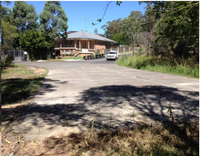
Figure 8 General view of the subject area facing south
