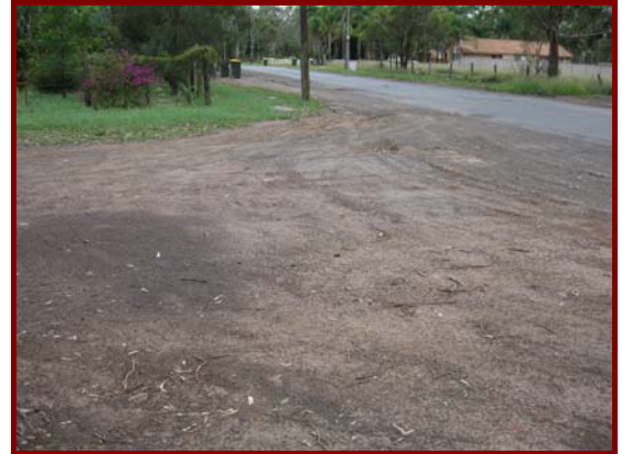
Figure 7. Example of exposed clay soils and ironstone, Crown Street facing east.
