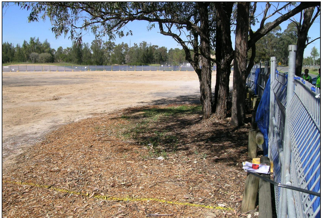
Photo 2-5 Proposed transformer location within the Fairfield RWTP
