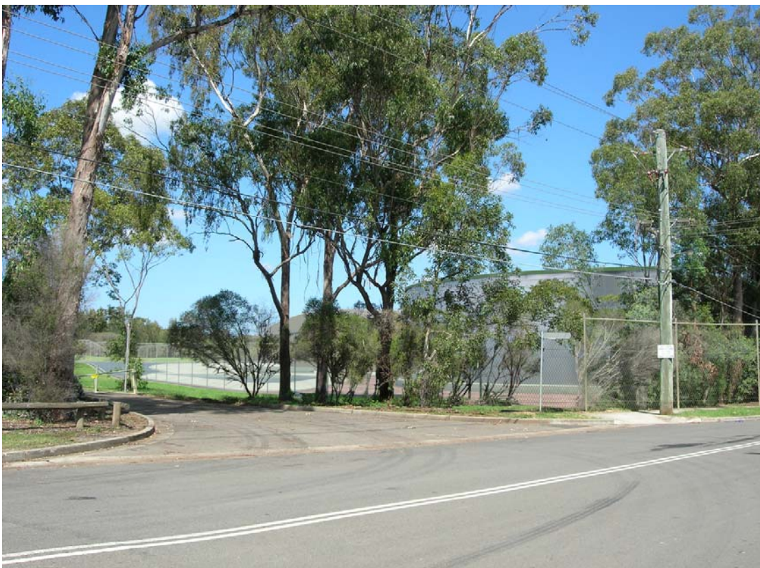
Figure 4-2 Revised visual photomontage of Fairfield water recycling plant from eastern boundary on North Street
