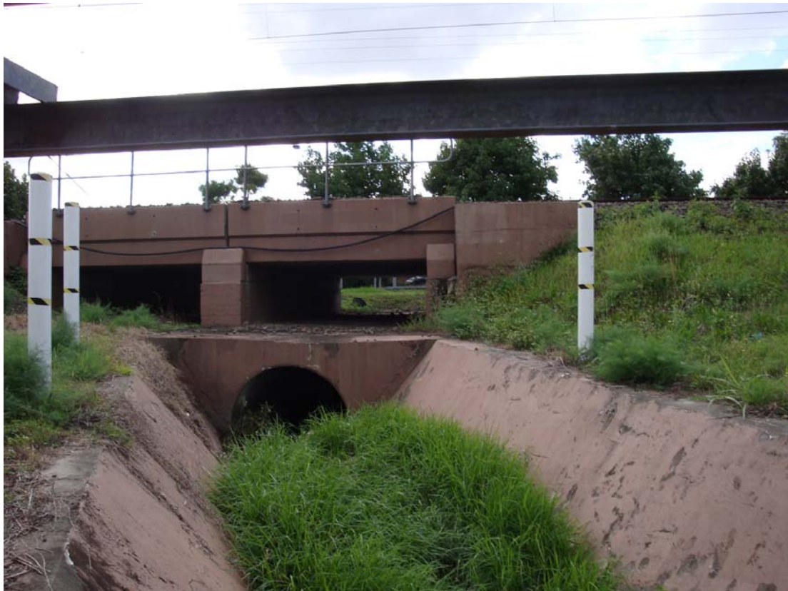
Figure 5-4 St Elmo's Drain underneath the railway line
