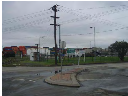
Plate 24: Shell Refinery, Rosehill. View faces southeast.
