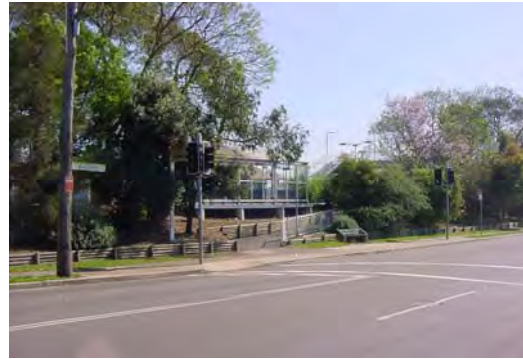
Plate 6: View of Yennora Railway Station. View faces northeast.
