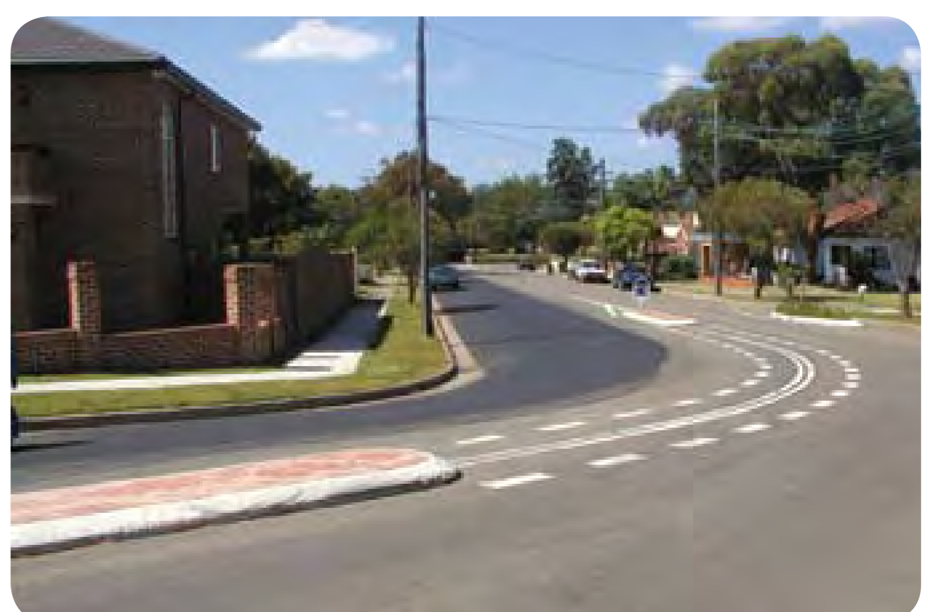
The final restoration of a trench in a roadway
