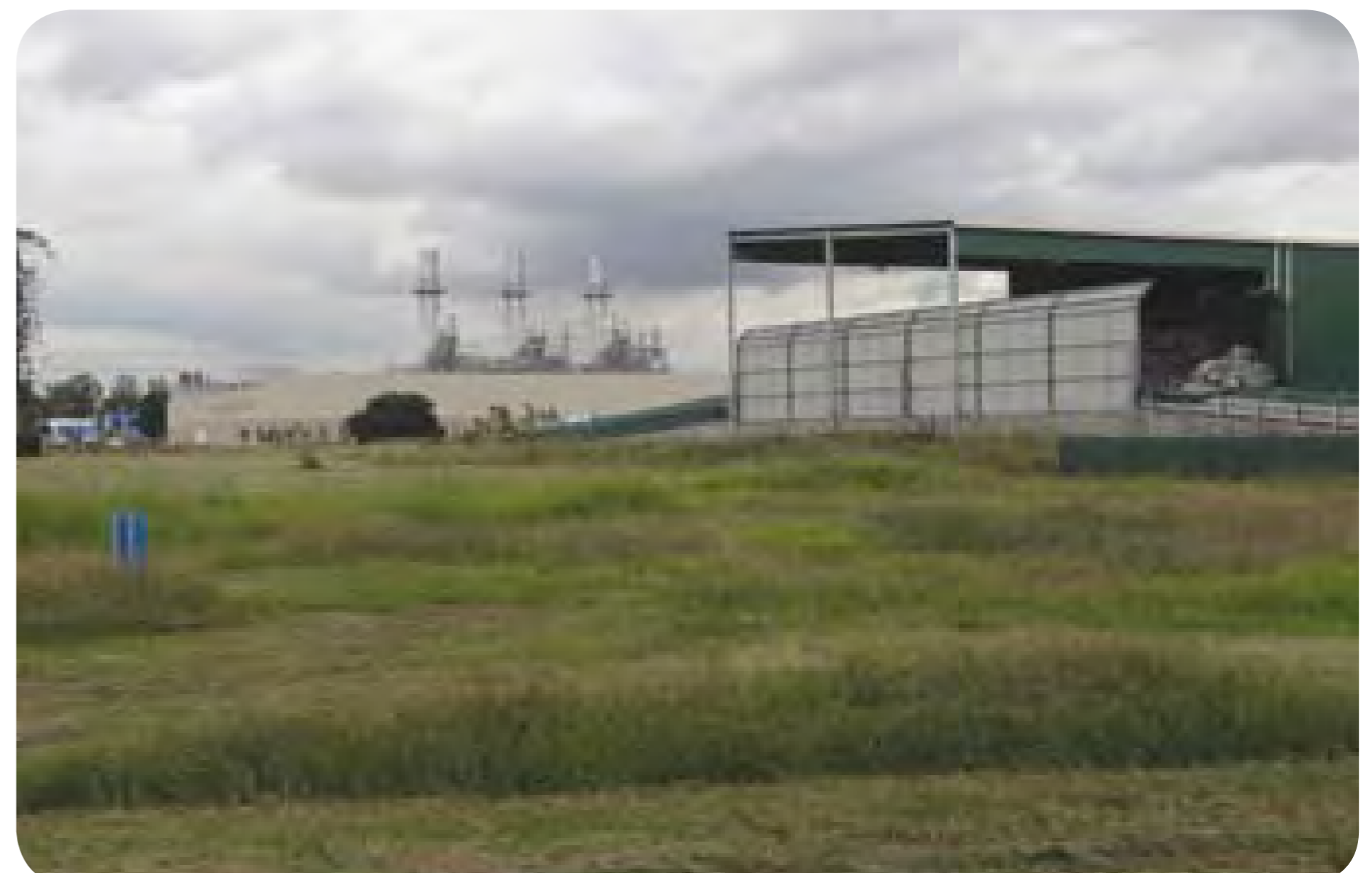
Marubeni Australia Power services and Visy Paper in Smithfield would be two of the customers that would use the recycled water
