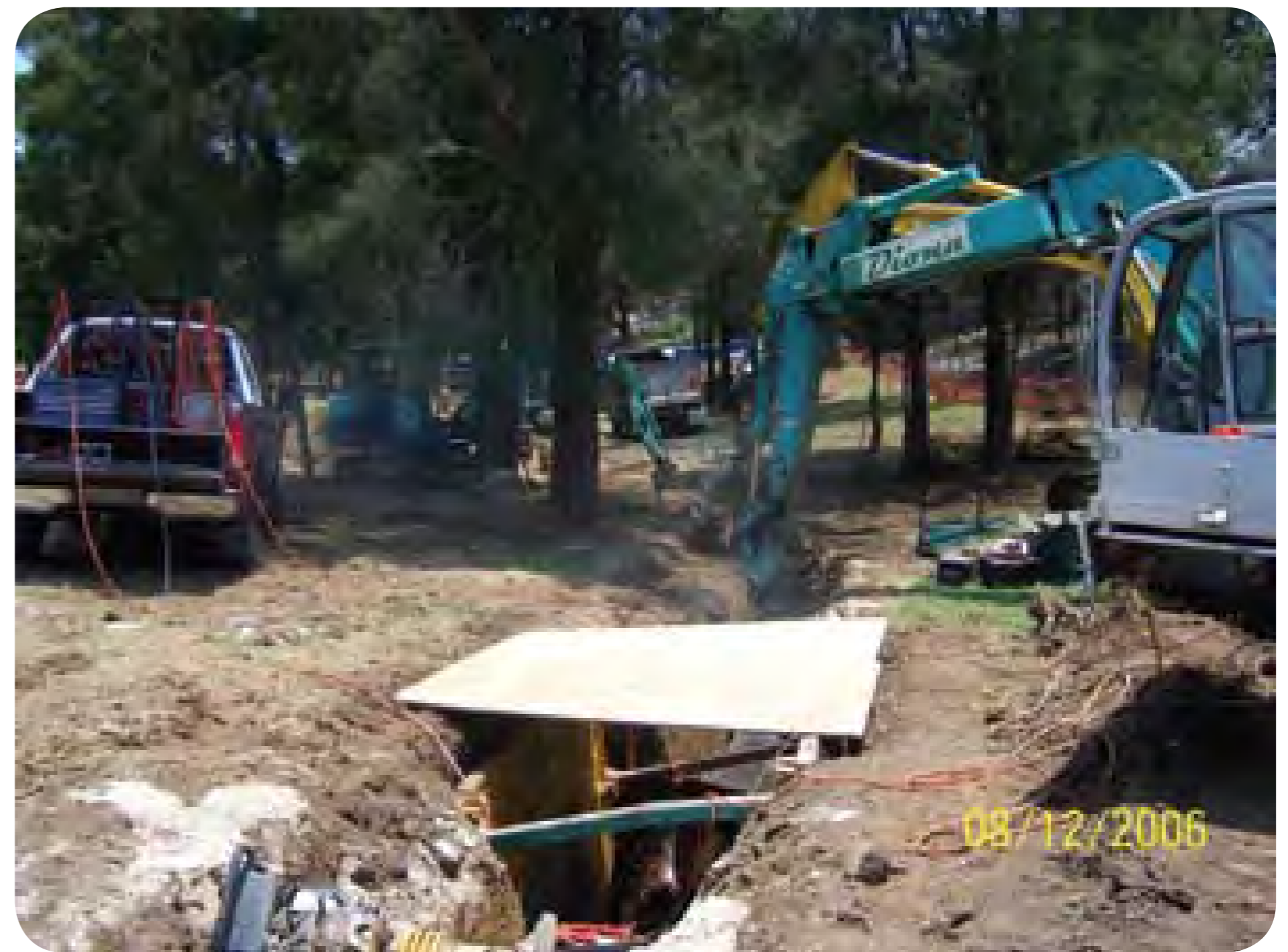
Trenching works through a public park
