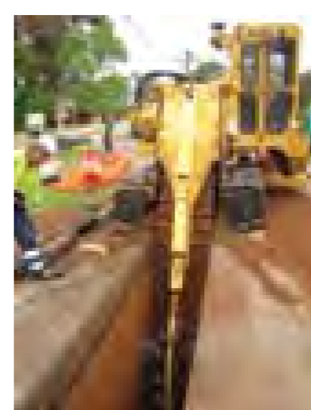
A trenching machine at work in a roadway
