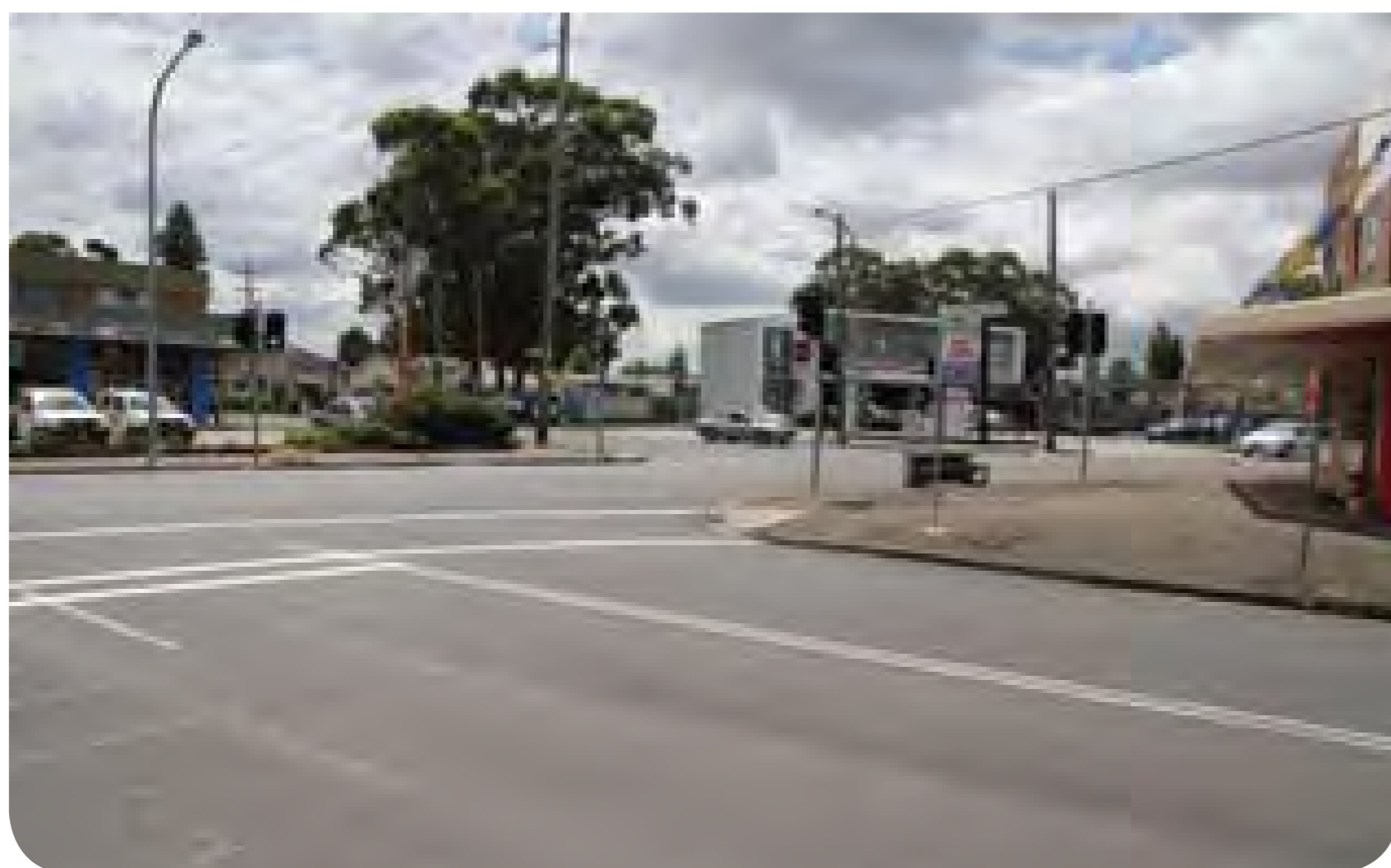
The proposed distribution pipeline would be installed underneath Fairfield Street from Crown Street in Fairfield East to Ellis Parade in Yennora using a cased bore to help minimise traffic disruption
