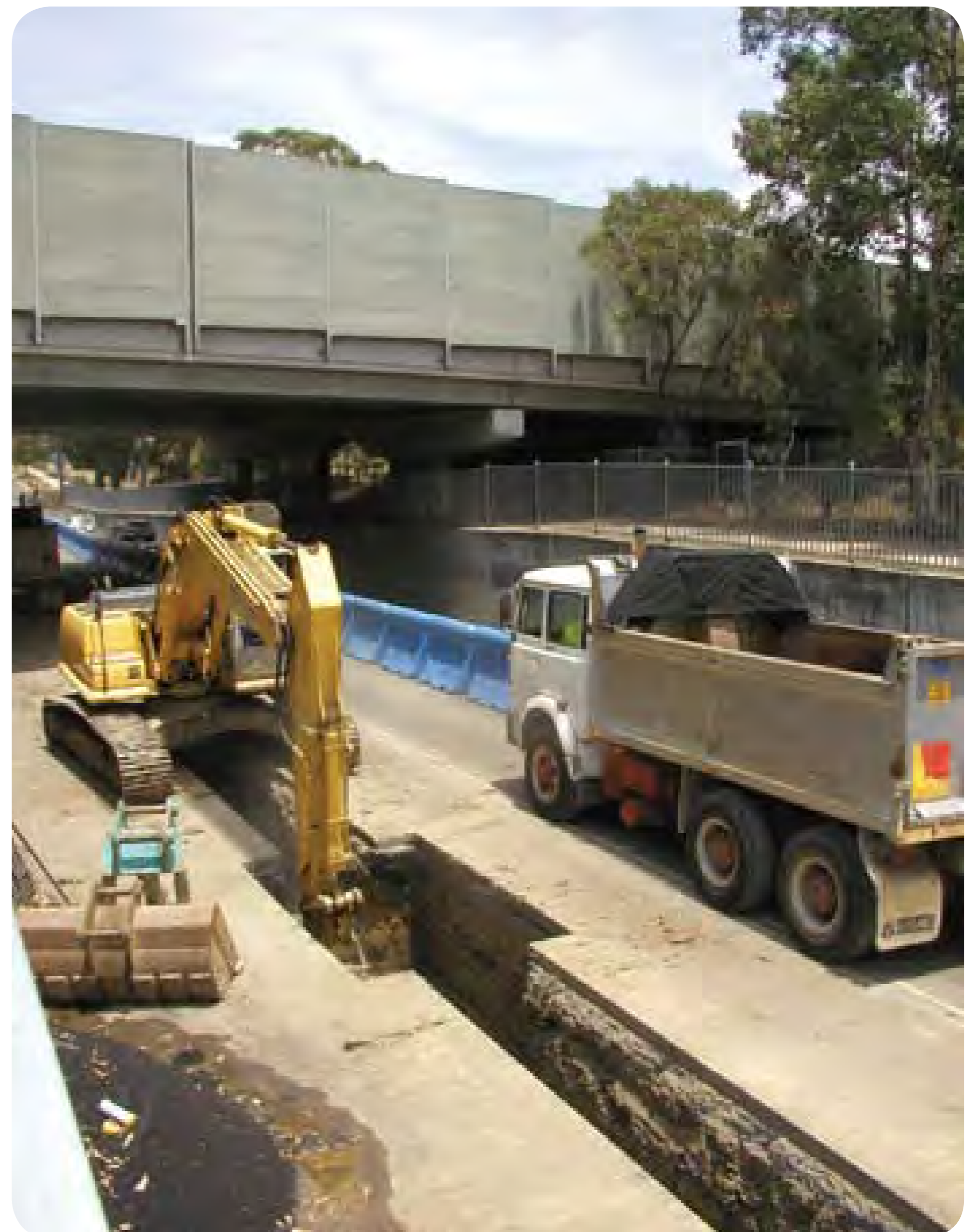
Trenching works in a roadway
