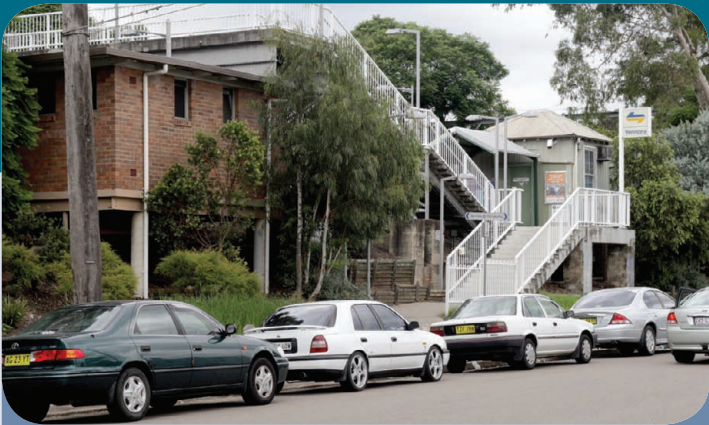
The proposed pipeline would be installed under the rail line beside Yennora Station using case boring to avoid impacts to the rail line and commuters.
