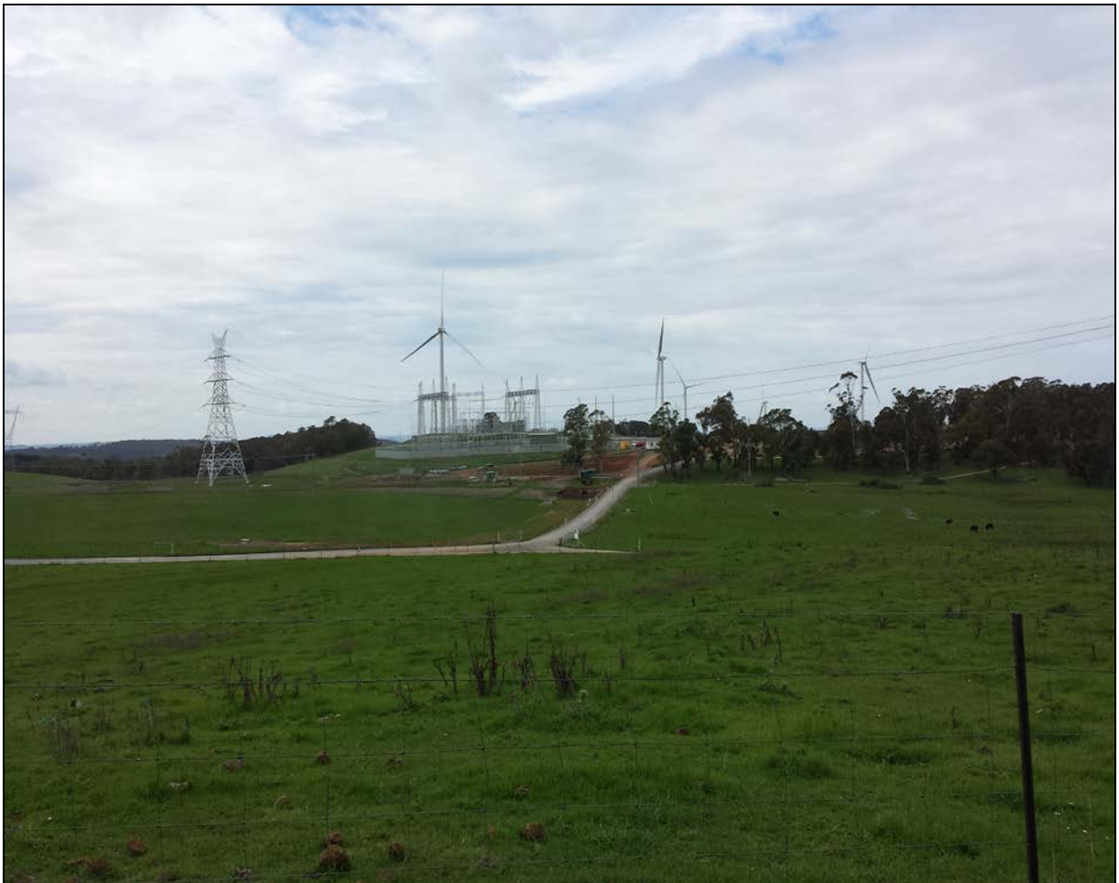
Figure 6: View towards the substation from the PW4 property (source: Department's site visit 9/4/14)).
