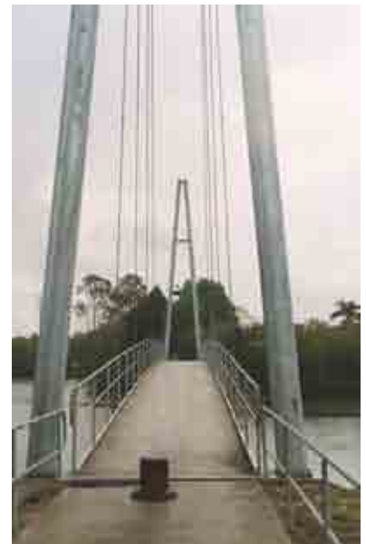
Pedestrian Bridge at Newee Creek
