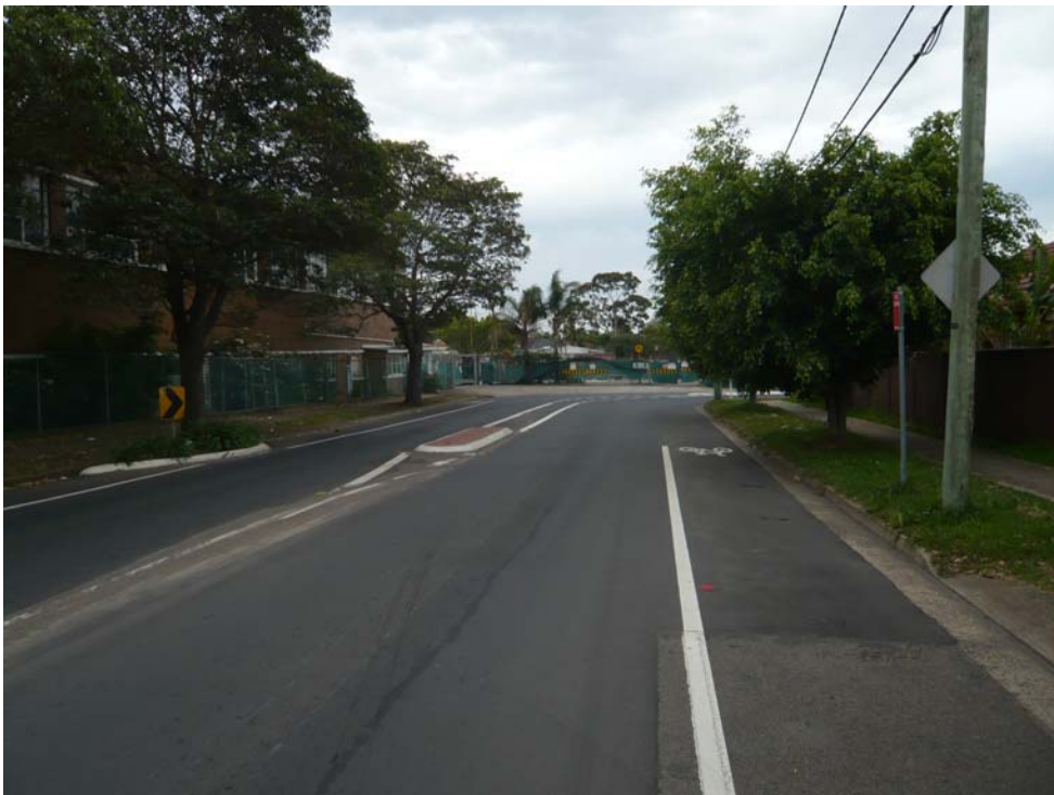
Reverse view looking east in Harp Street on approach to the sharp bend (which will be eliminated and replaced with a cross junction).
