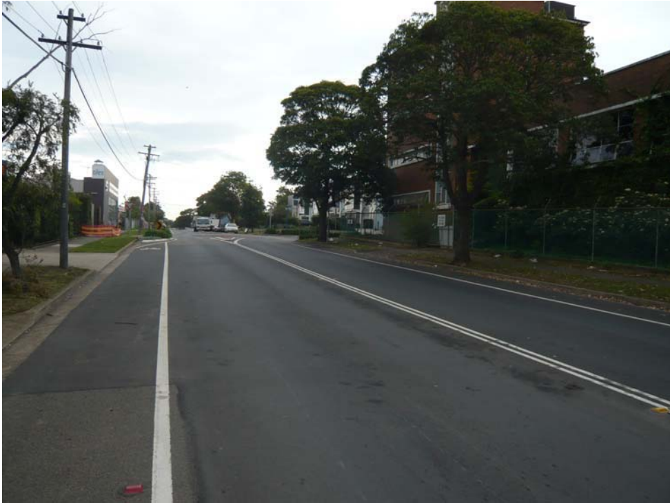
View looking west in Harp Street adjacent to the site with the Charlotte Street roundabout in the distance.
