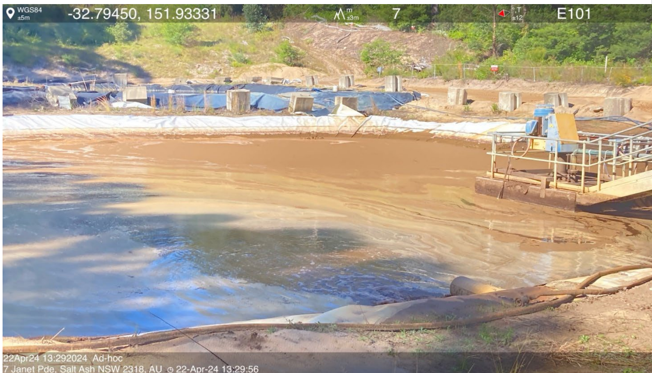
Lower retention basin
