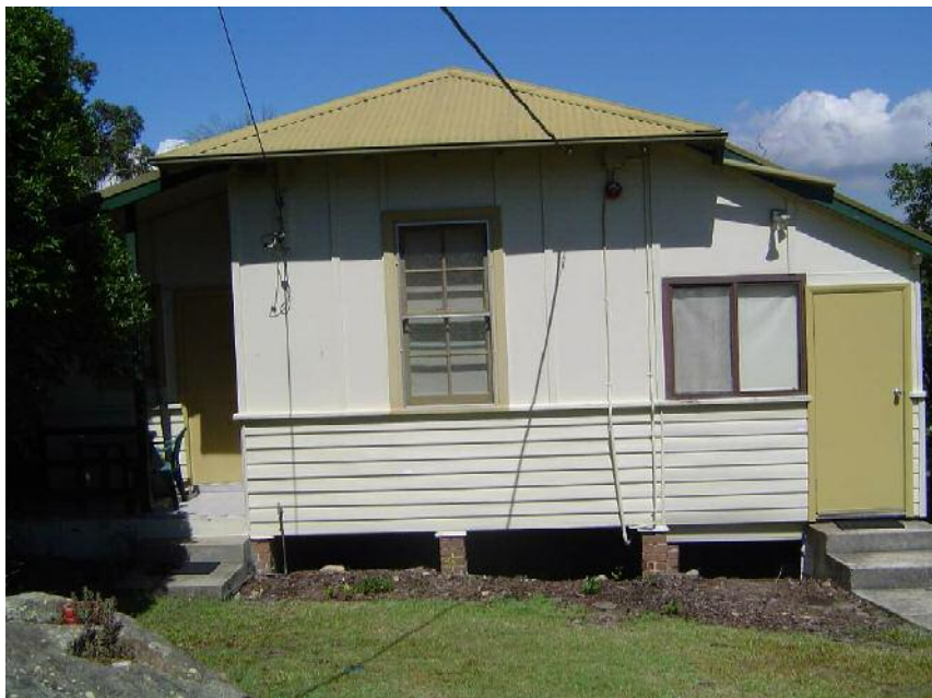
Figure 12 - Photograph of Garden Cottage an example of the former staff accommodation viewed from the east showing in-filled verandah at right. Noel Bell, Ridley Smith & Partners - 2006.
