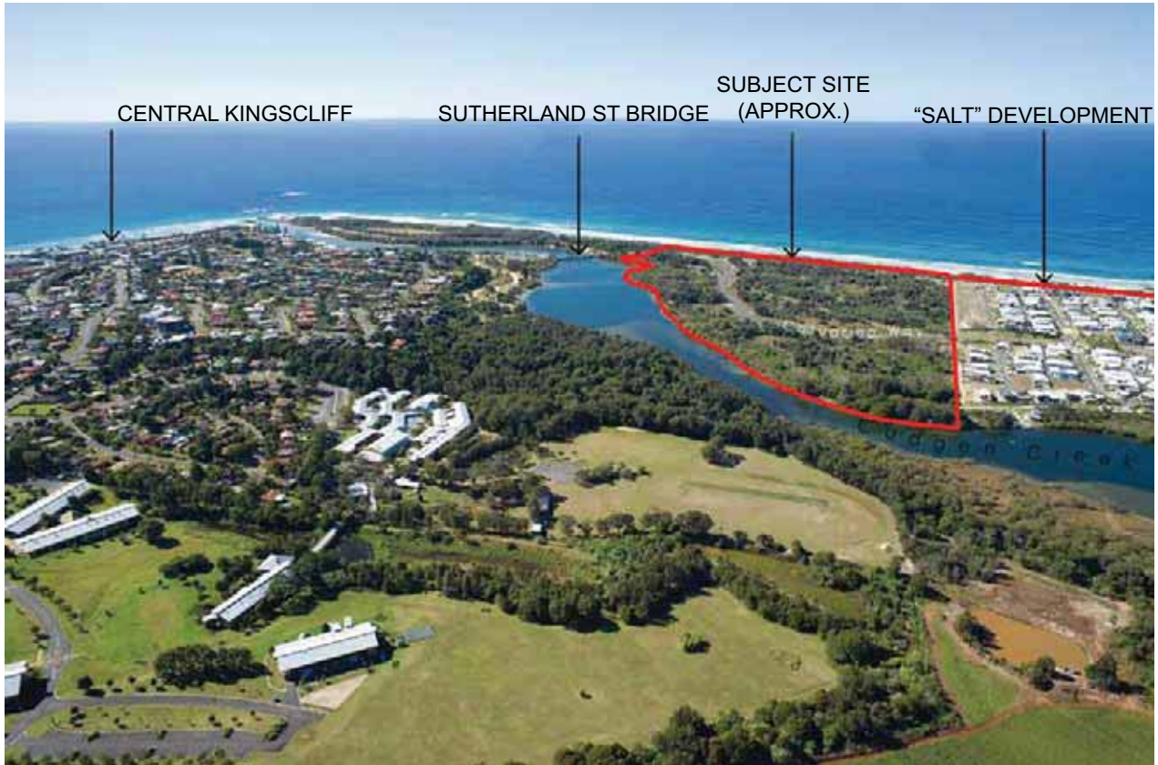
AERIAL PHOTOGRAPH VIEWING EAST SHOWING SITE CONTEXT
