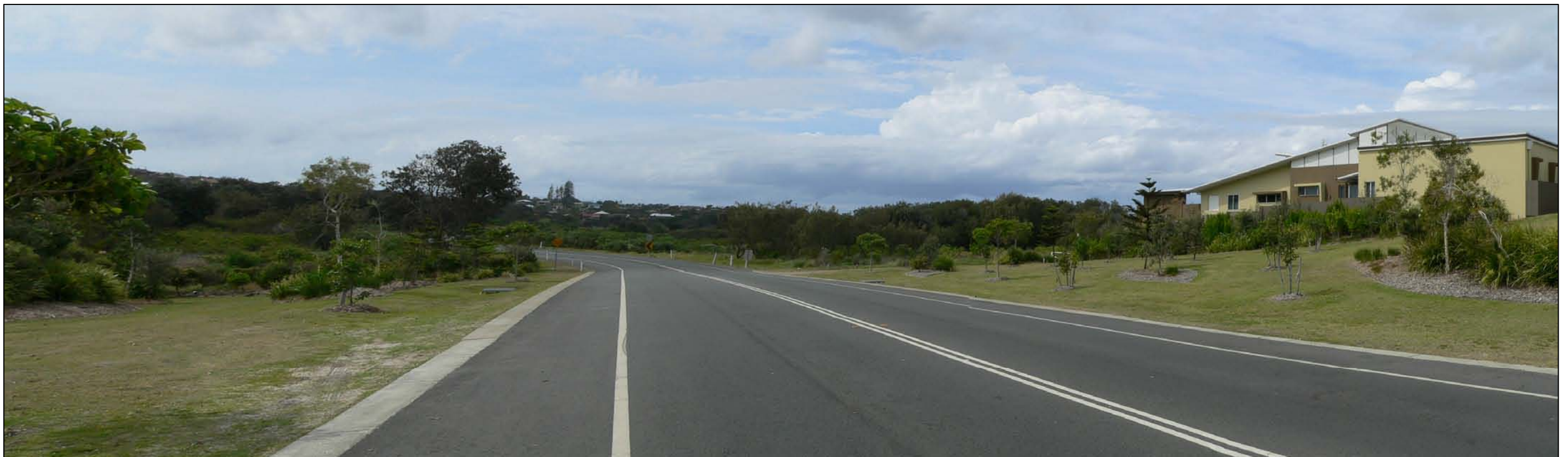
Figure B2 - View north along Casuarina Way, with Salt development in the foreground, the site in the mid-ground, and the established Kingscliff settlement in the background.
