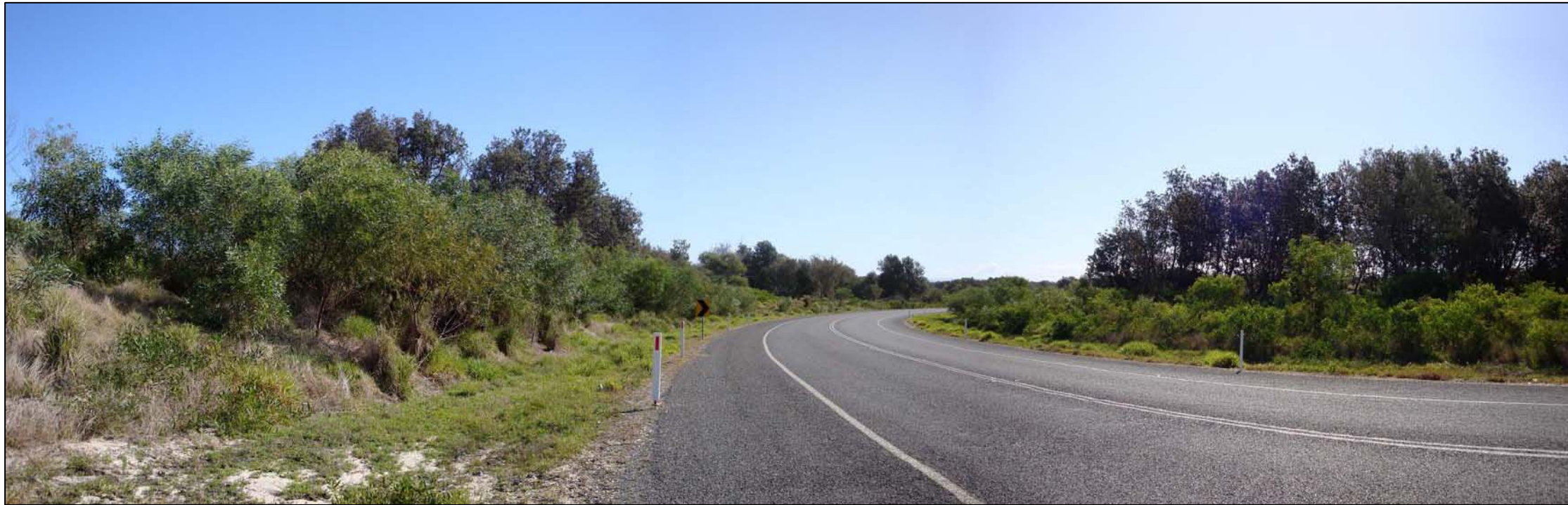
Figure C1 - View from PP01 - BEFORE
