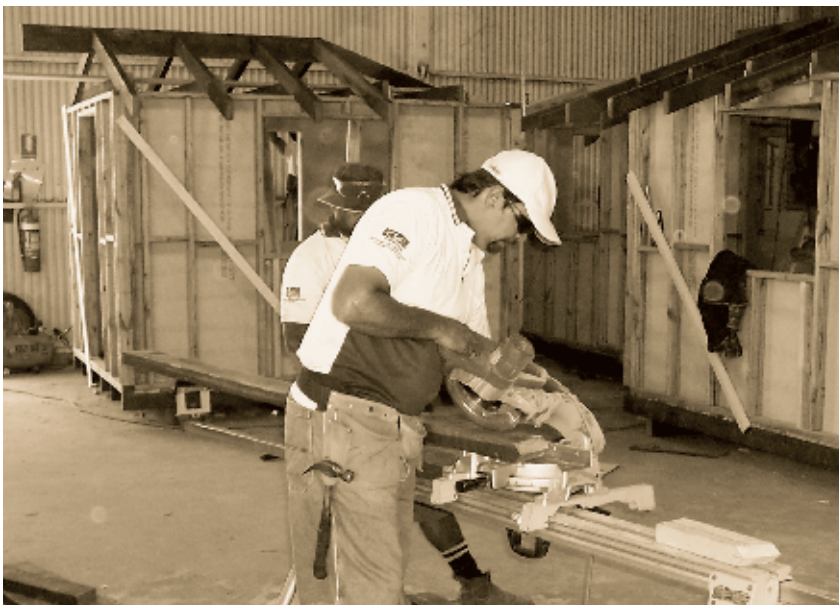
Arnold McGrady cutting angles for the roof construction on the Boggabilla/Toomelah Project.
