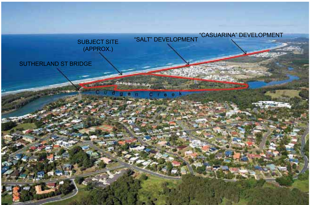
AERIAL PHOTOGRAPH VIEWING SOUTH EAST SHOWING SITE CONTEXT
