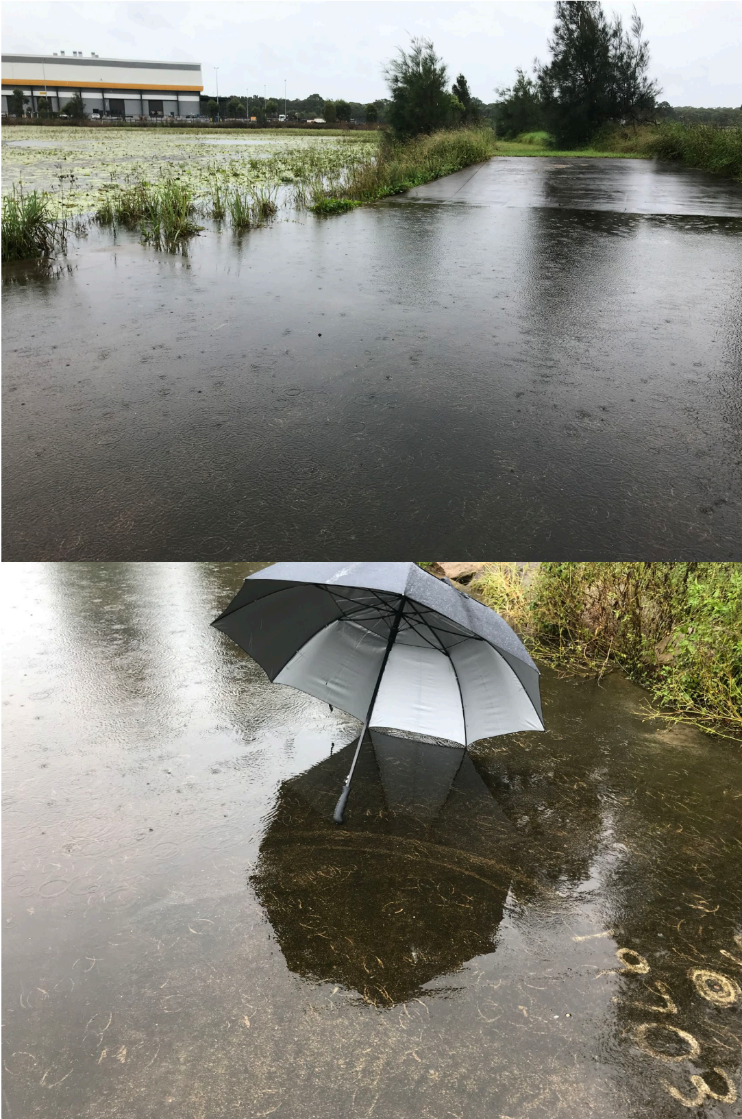
Plates 6.3 & 6.4 – Spillway at 22 March 2021. 330mm of rainfall in 5 days prior, ~10mm depth over spillway – umbrella used for water depth perspective. Clear water quality.
