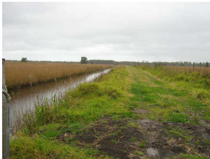
Plate 4 – Spoil embankment track
