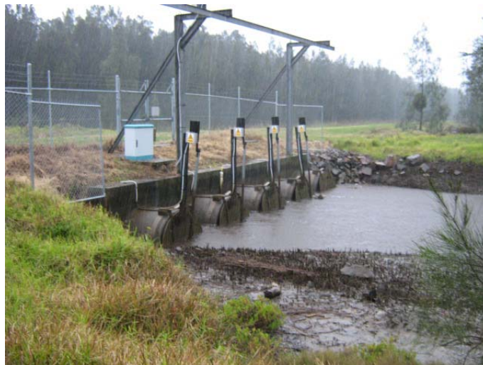
Plate 6 – Five 1500mm Pipe Crossing
