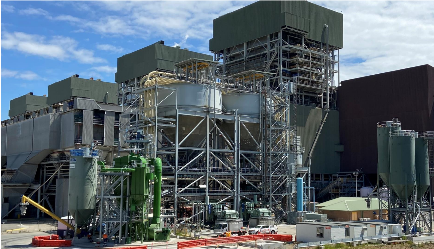
Figure 4 Existing Daracon Facility Including Classifier (Left) and Storage Silos (Right)
