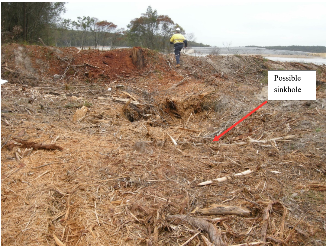
Figure 3.6 View of possible sinkhole location
