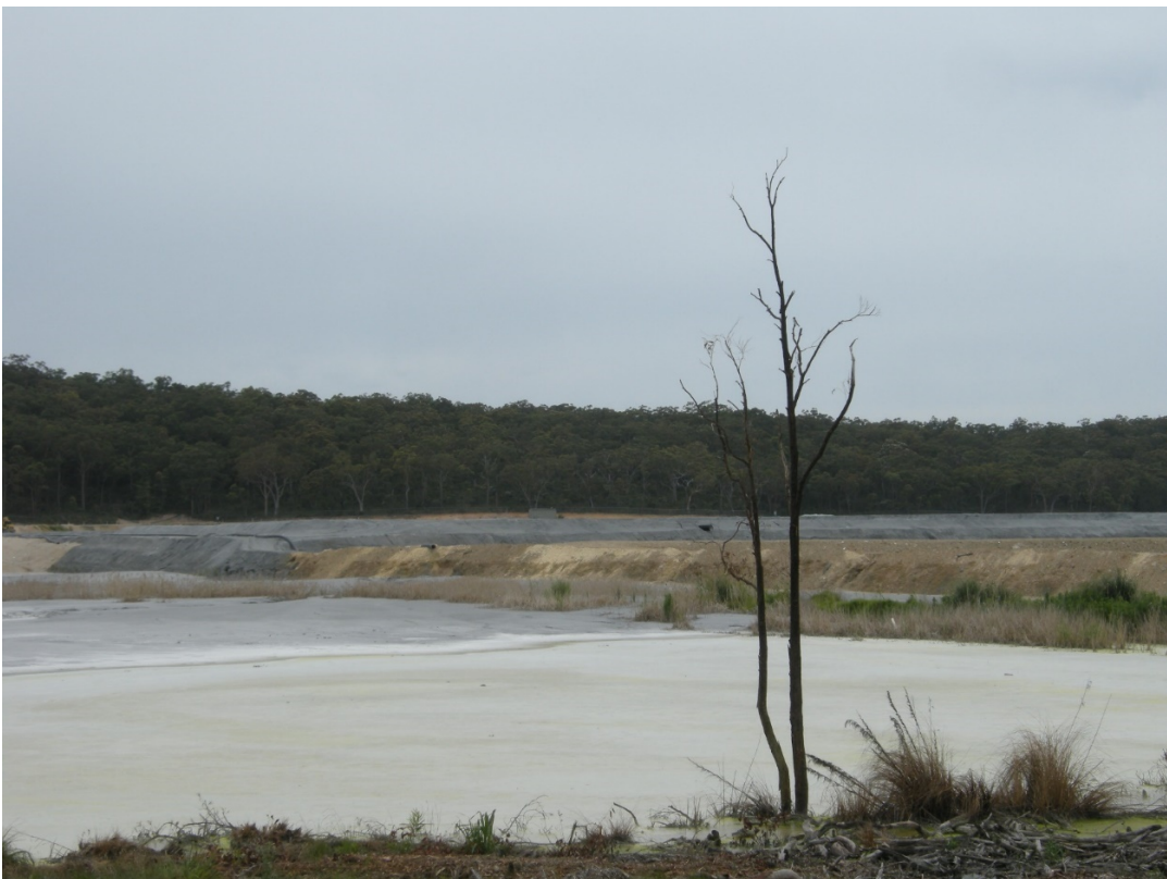
Figure 3.2 View of downstream side of cell at existing facility
