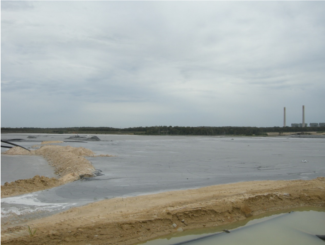
Figure 3.5 View showing extent of existing facility looking towards station
