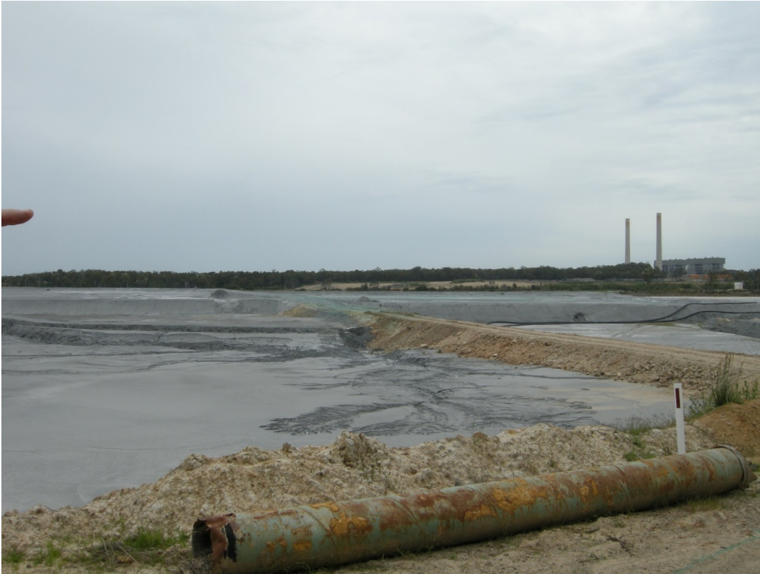
Figure 3.3 View of existing facility looking towards station
