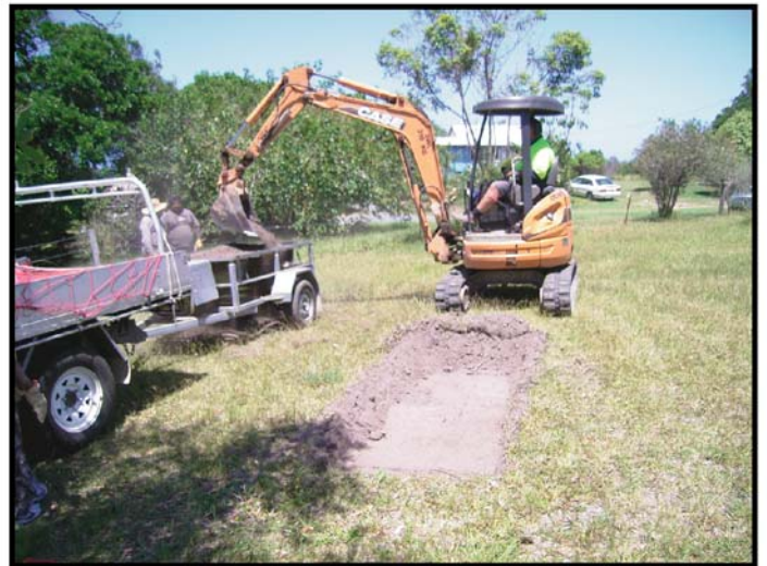
Plate 4. Excavated sediments placed directly on mechanically-agitated sieve (TP B/6).
