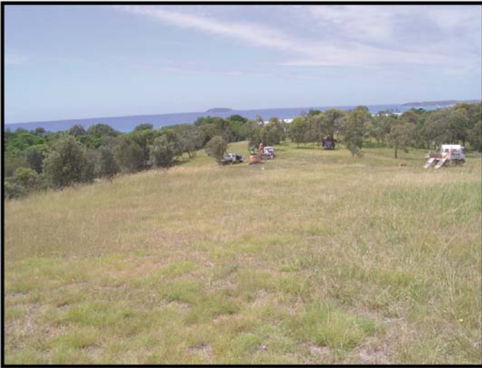
Plate 1. View south from ridge summit (occupied by an existing house) towards the investigation area. Test excavations in progress.
