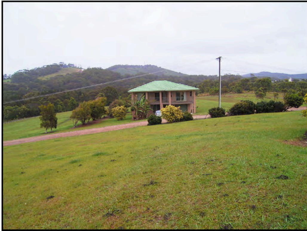
Plate 5. View from levelled ridge knoll across moderate gradient slopes in the south-west part of the study area
