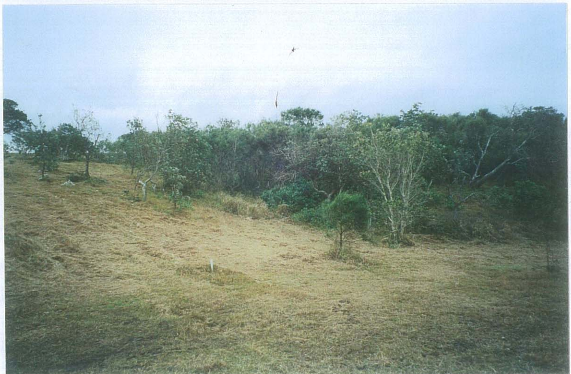
View looking westwards into the southern end of the Zone steep erosion gully with slumping sides
