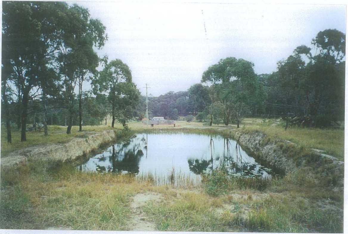
Water storage pond on main ridge top. Excavation at least 2½ m deep.
