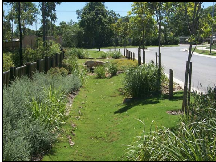
Figure 4-2 Vegetated swale (DEC, 2004a)
