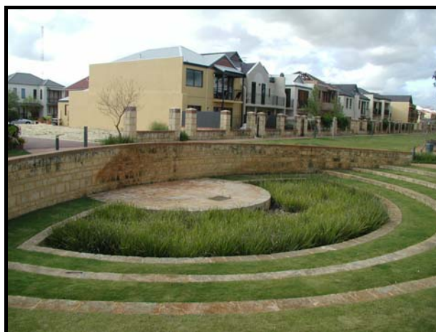
Figure 4-3 Bioretention basin with central filter (ARQ Draft, 2004)
