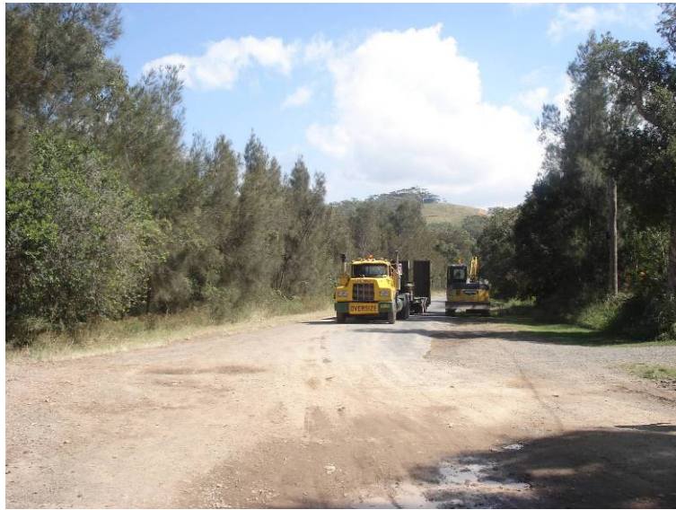
View west from the south-western corner toward the sealed portion of Hearn's Lake Road.
