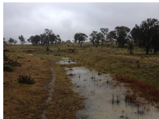
Plate 4. Disturbance associated with dam construction
