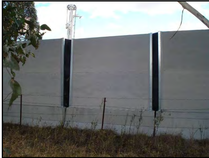
Plate 4. Noise Mitigation Barriers
