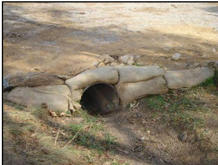
Plate 6: Erosion and Scour Control Structure
