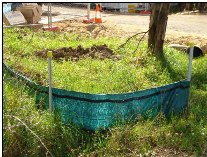
Plate 7 Sedimentation Control Structure
