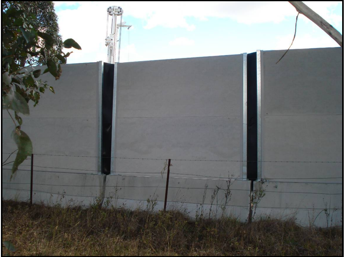
Figure 6 Noise Mitigation Barriers
