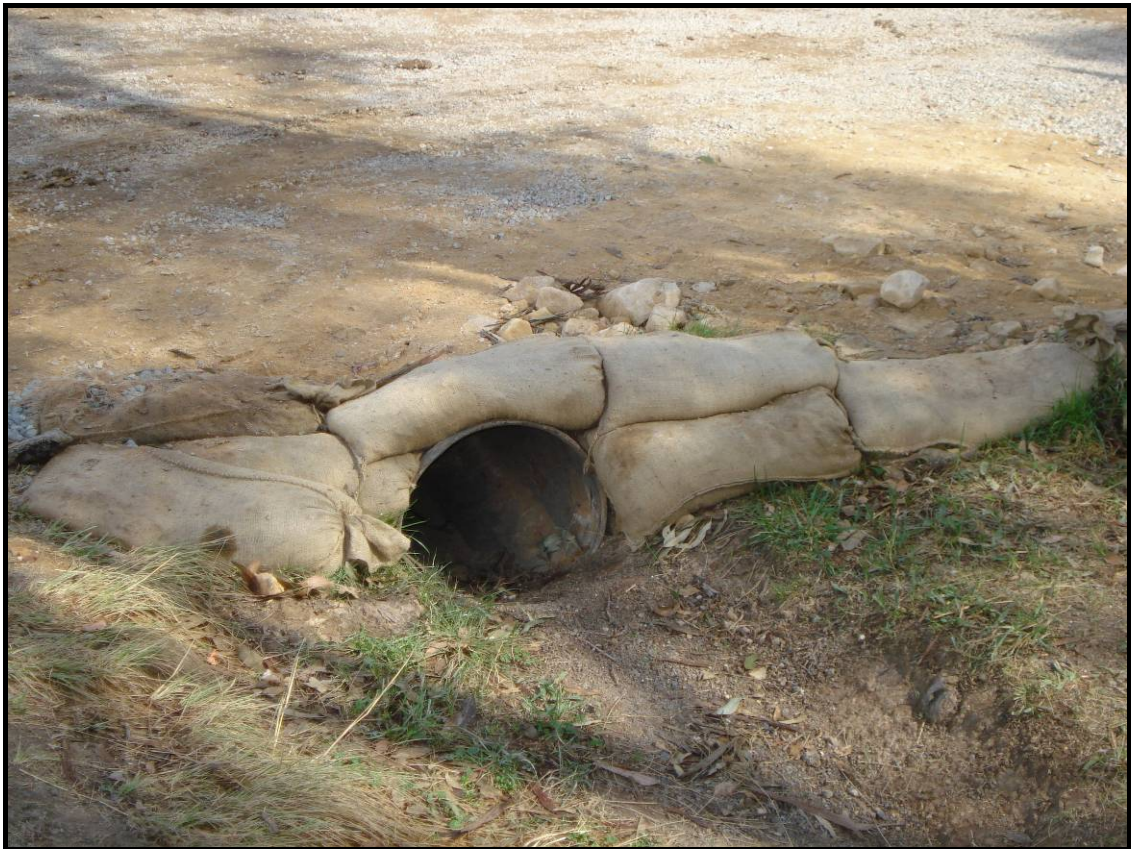
Figure 9 Erosion and Scour Control Structure
