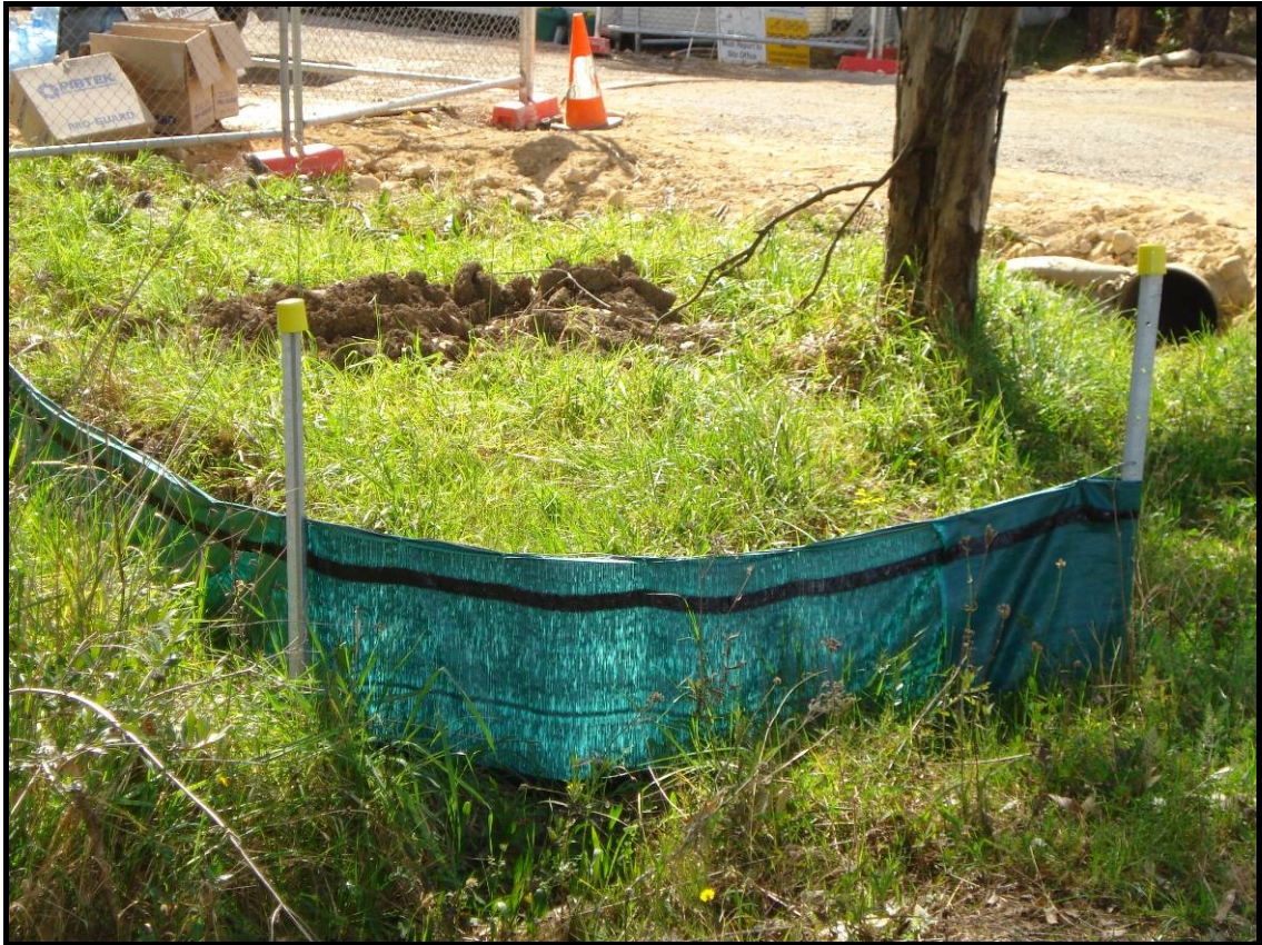
Figure 10 Sedimentation Control Structure
