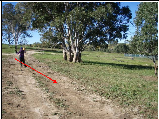
Plate 6 :newly graded track and location of disturbed site 52-2-0021
