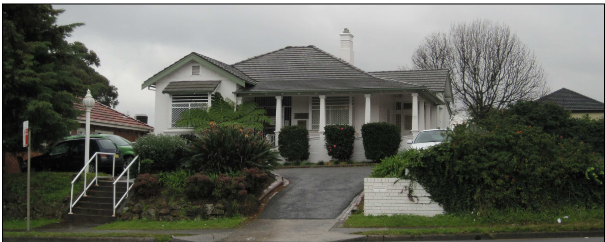
Figure 25: Local Heritage Item - 366 Crown Street
