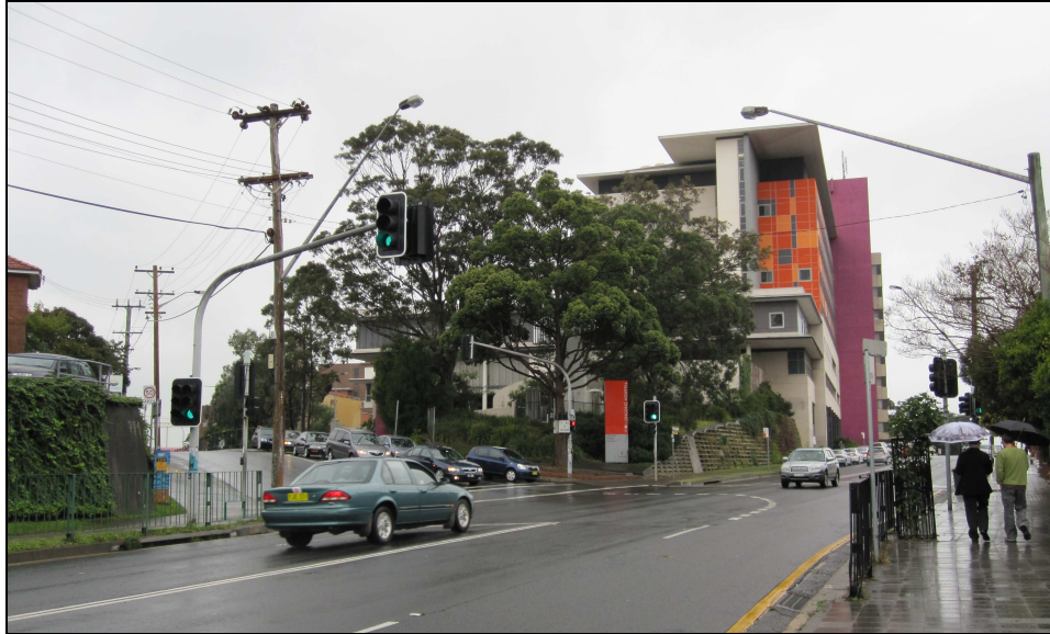
Figure 18: Wollongong Public Hospital– easterly view
