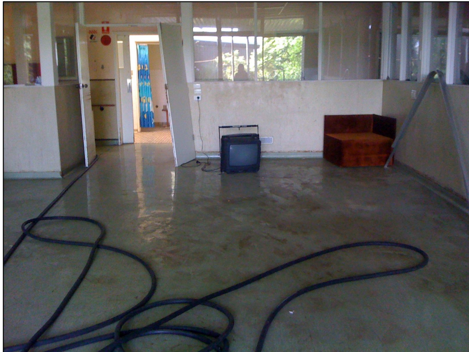
Plate 3 – Common room within the nursing home building (12/2/2010).
