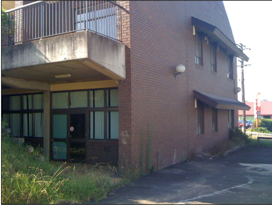
Plate 5 – Western side of nursing home building showing the balcony. Frame looking southeast (12/2/2010).
