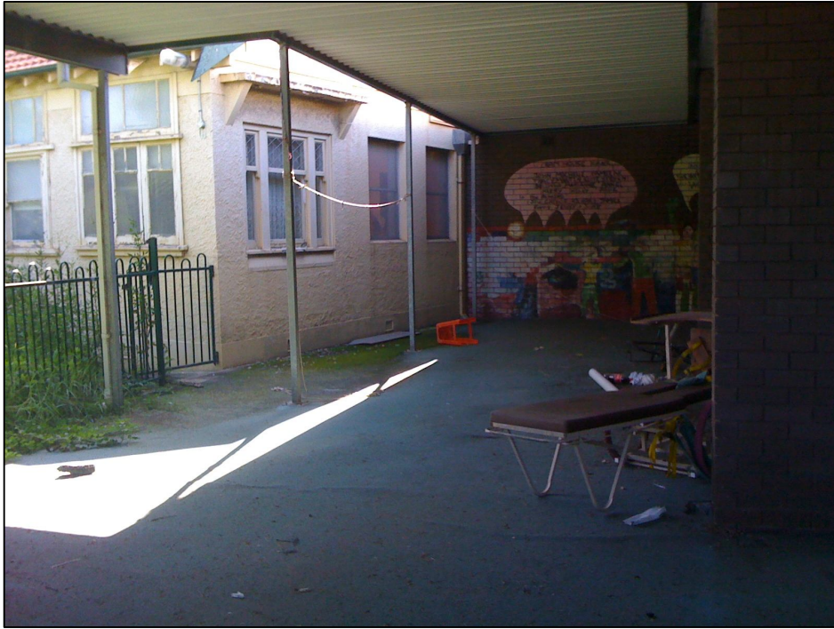
Plate 9 – Residential dwelling connecting to the nursing home building at its northeastern corner. Frame looking northeast (12/2/2010).
