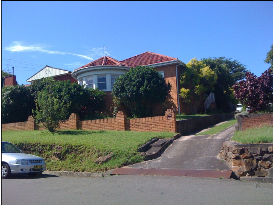
Plate 21 – Residential dwelling at 9 Urunga Parade. Frame looking southeast (12/2/2010).
