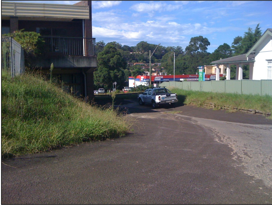
Plate 7 – Southwestern portion of the site (364 Crown St) showing mounded soil to the left of frame and a retaining wall garden bed along the western boundary. Frame looking southwest (12/2/2010).
