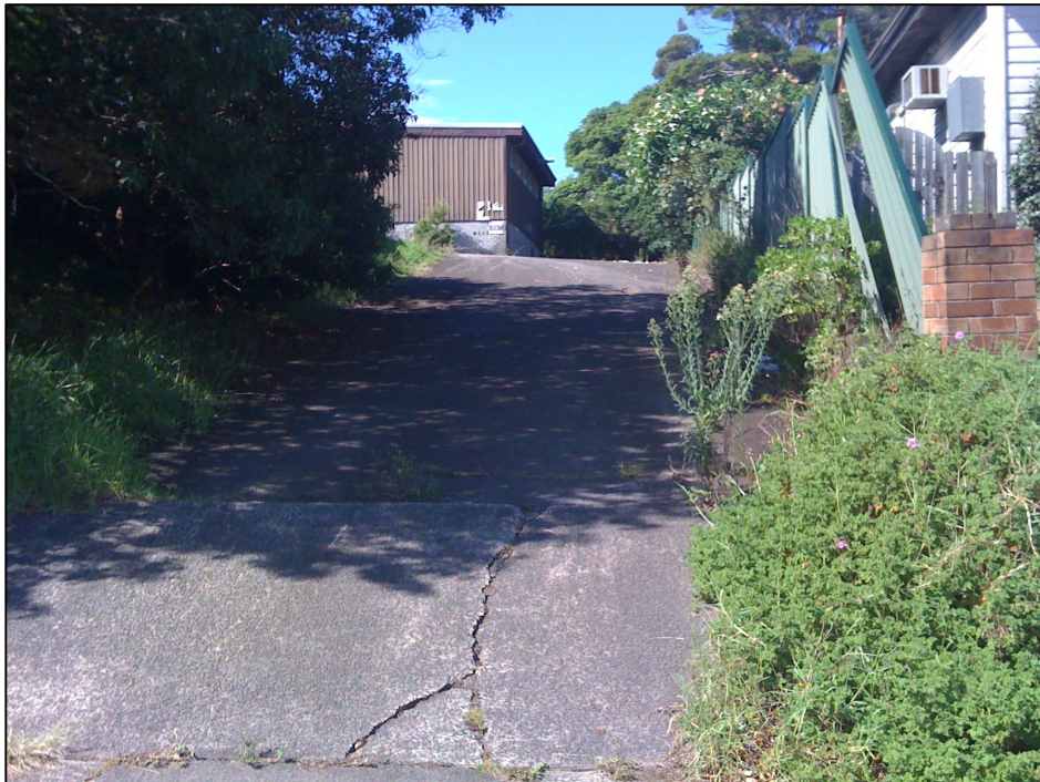
Plate 18 – Driveway entrance from Urunga Parade. Frame looking south toward the site (12/2/2010).
