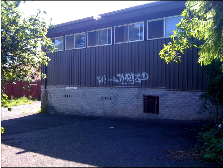
Plate 13 – Hydrotherapy pool building located to the northeast of the residential dwelling. Frame looking northeast (12/2/2010).
