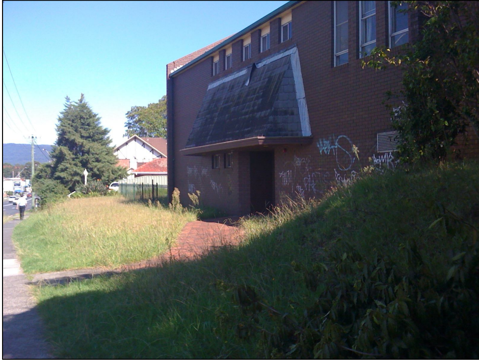
Plate 1 – Nursing home building fronting Crown Street. Frame looking northwest (12/2/2010).
