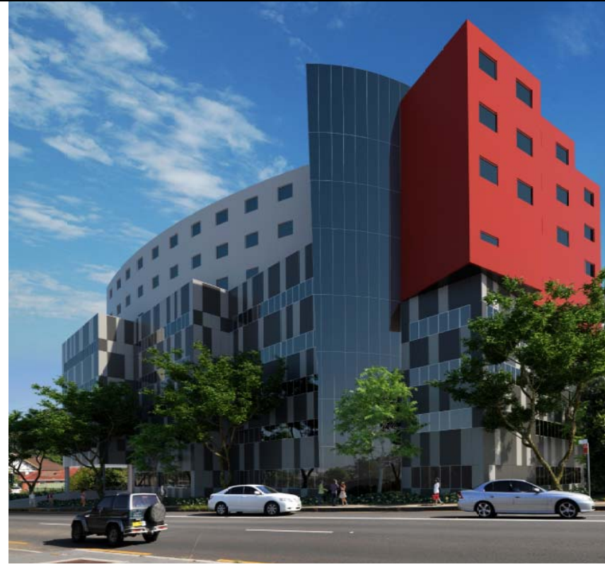
Figure B: Visual representation as submitted with Environmental Assessment to Crown Street looking west
