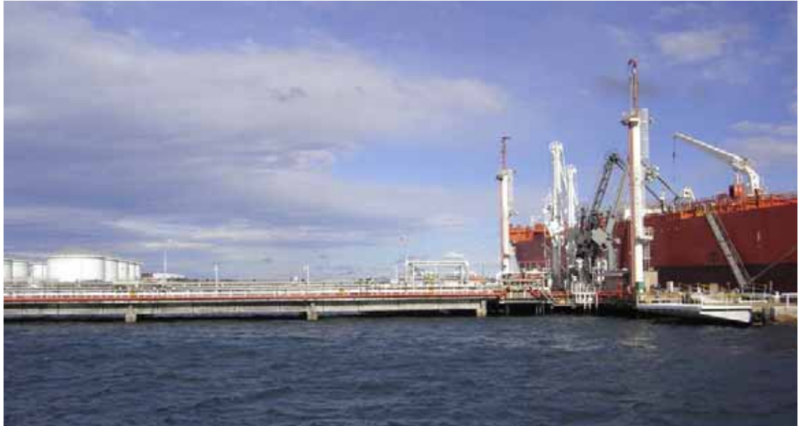
■ Figure 4-4 Existing BLB1 bulk liquids berth
