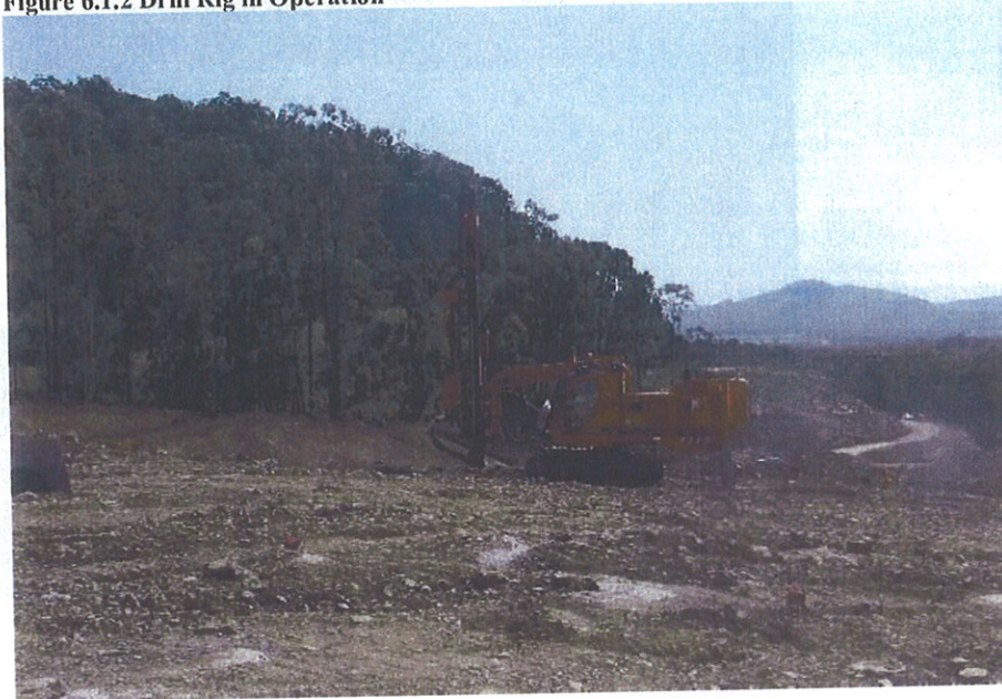
Figure 6.1.2 Drill Rig in Operation
