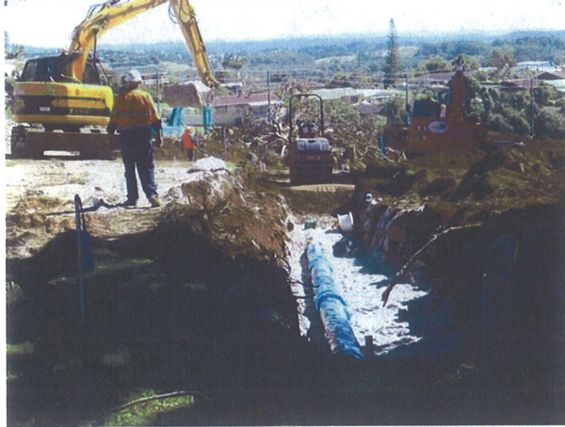
Figure 4.8.2 Underground Watermain Installation
