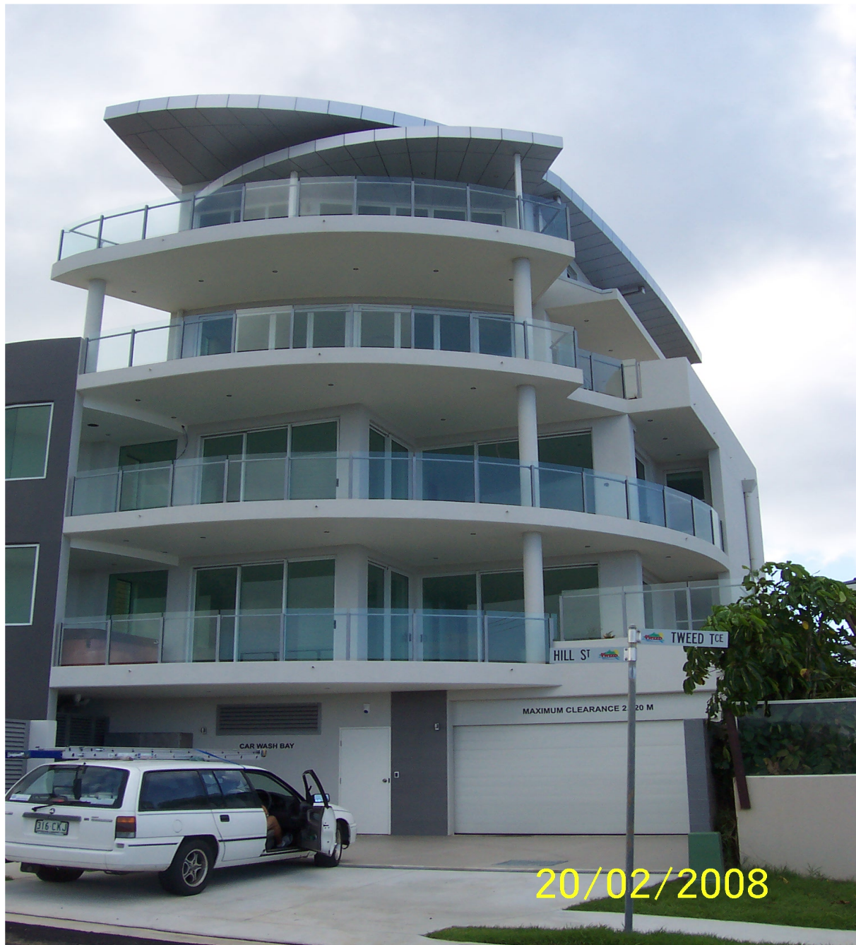
Figure 5 – Adjoining 5 storey residential flat building located on the corner of Hill Street and Tweed Terrace. This development shares the rear boundary with the subject site.
