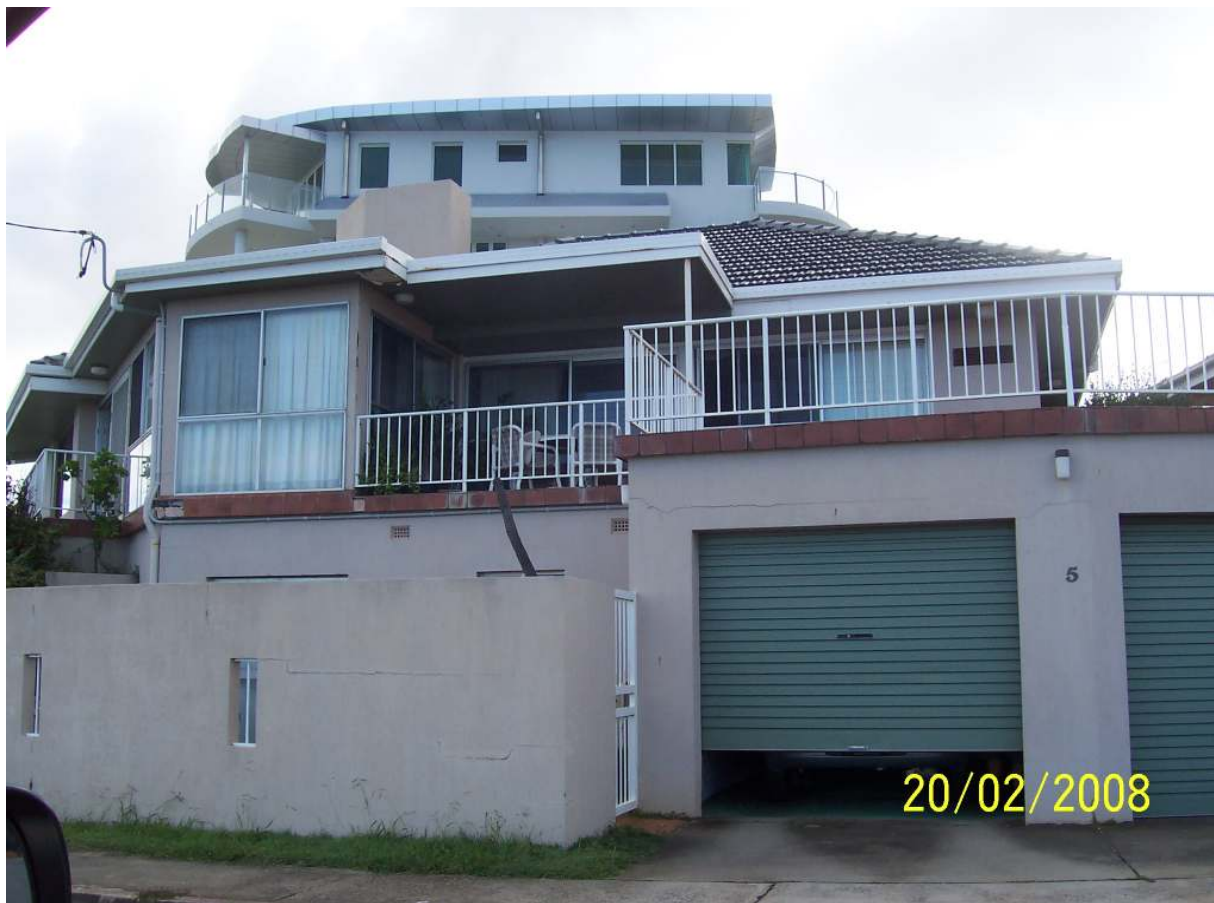
Figure 4 – Existing 2 storey concrete rendered dwelling on the site
