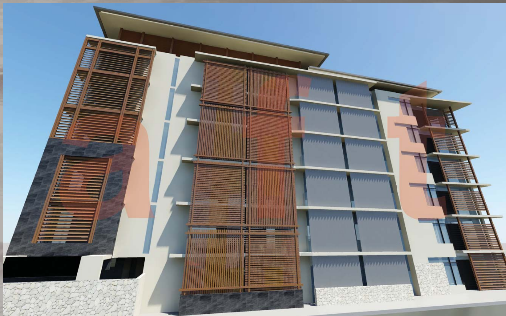
view of south-west facade
