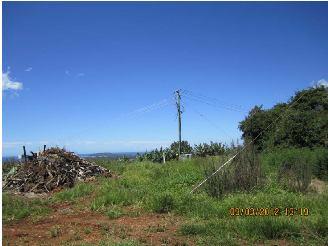
Figure 10 View from within the proposed TCC site looking north east toward the coast. Note pile of demolition rubbish in foreground
