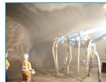
Additional roof support - shotcrete
