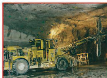
Installing rock bolts to provide roof support
