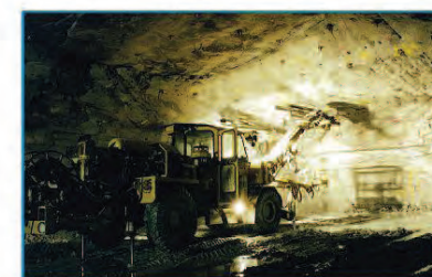
Drilling blast holes
