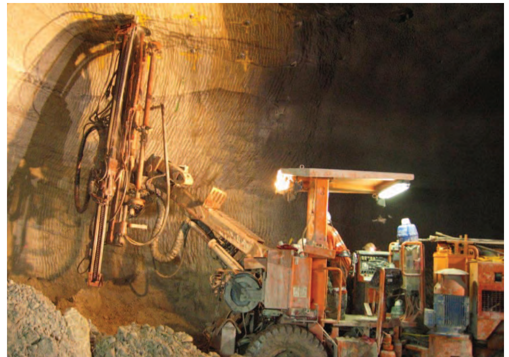
Installation of rock bolts
