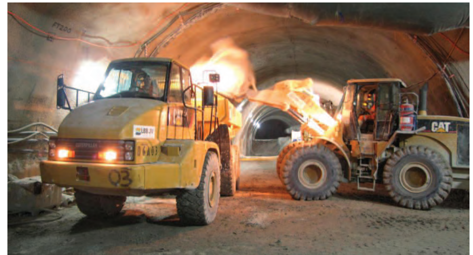
Mucking (removal of blast material)
