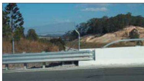
Illustration 95: This design detail has successfully integrated a safety barrier and bridge parapet (source: RTA 'Bridge Aesthetics', p 43)
